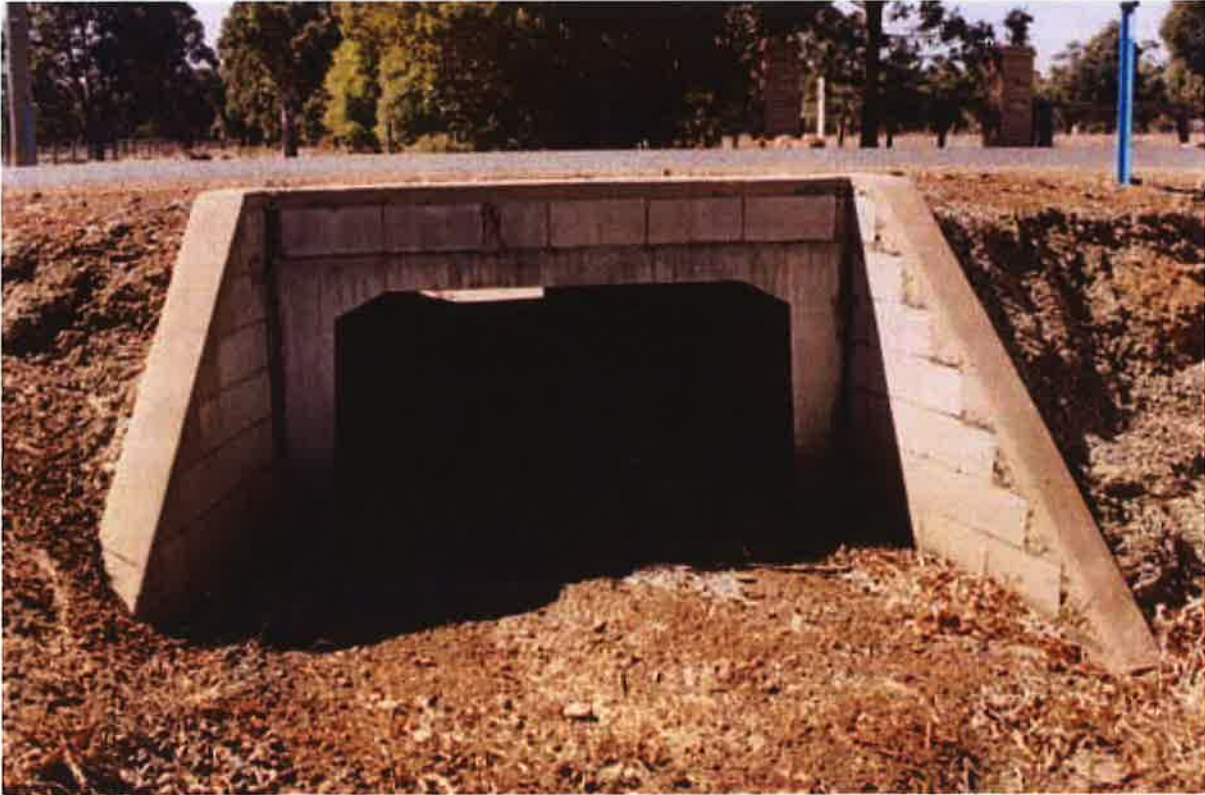
Drainage Culvert under Briggs Road
