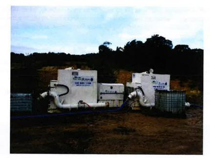
Plate 1: Water Treatment Dosing System at Shale Road
