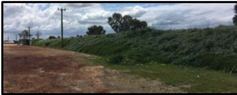
Figure 5: Existing 2.5m earthen bund
