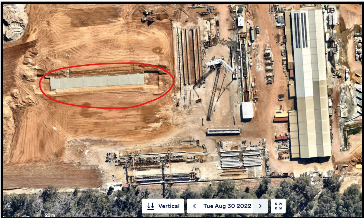
Image 7: 30 August 2022. Note new stressing bed being built with no Shire or DWER approval. Located close to the western boundary, and orientated in such a way that noise is directed in an east west direction.
