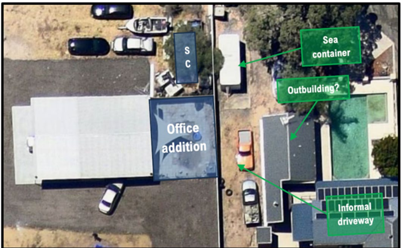
Figure 8: Development adjacent to the neighbours outbuilding and sea container
