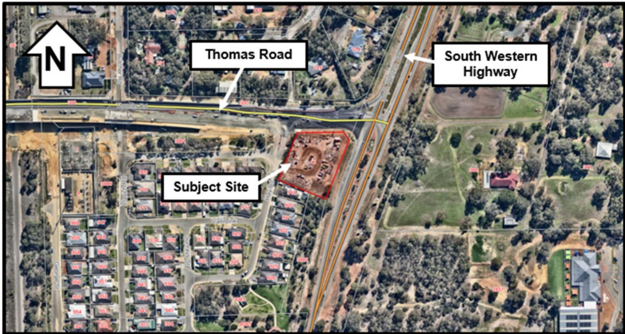
Figure 1: Aerial image of the locality
