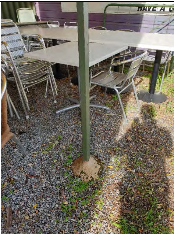
Steel section patio tube posts
