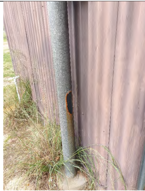
A large hole in what appears to be a ventilation stack
