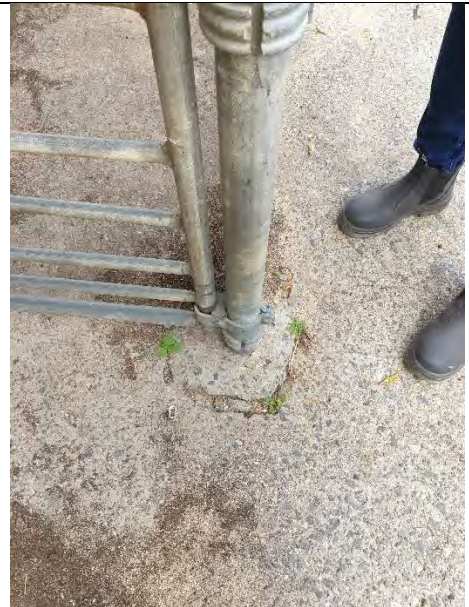
It appears new posts have been installed with new footings
