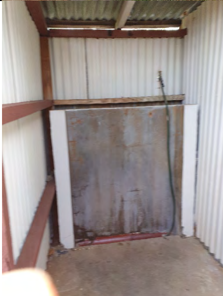
Concrete wall type urinal with hose attachment as flush
