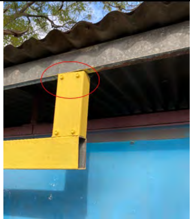
Cantilevered connection to building E
