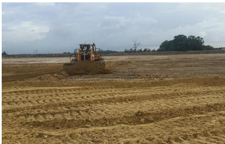
Plate 4: Final landforming post mining using a dozer
