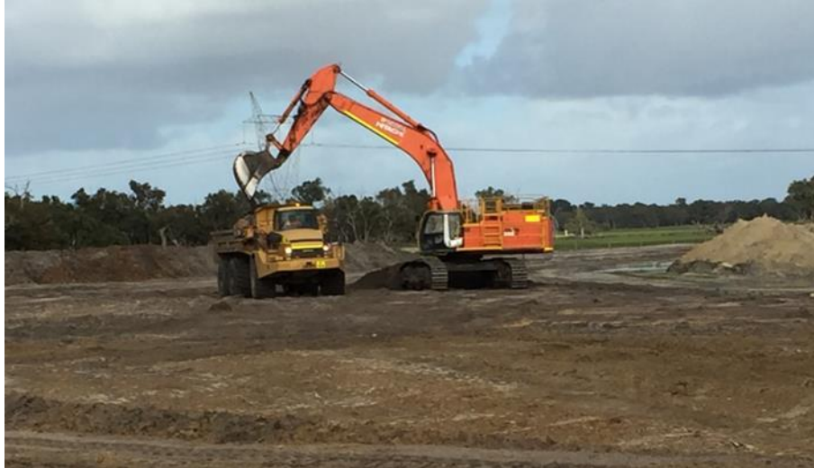
Plate 2: Stripped topsoil removal to stockpile
