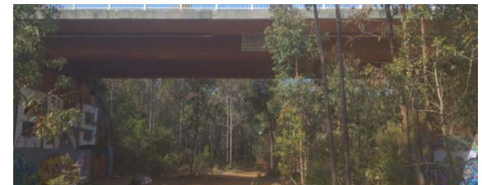
Existing Nettleton Road Underpass
