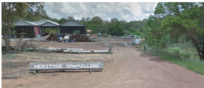
Jarrahdale Heritage Mill
