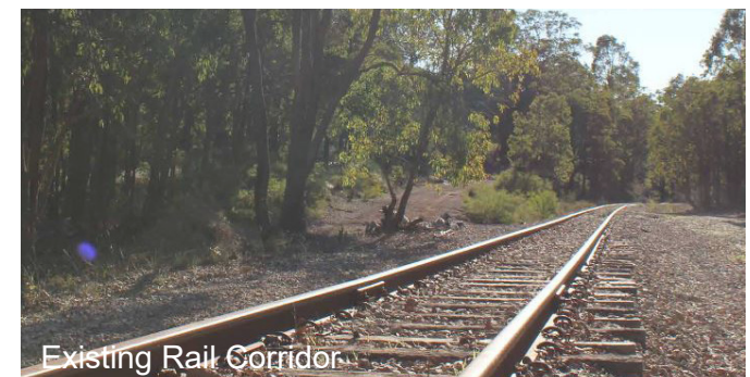
Existing Rail Corridor
