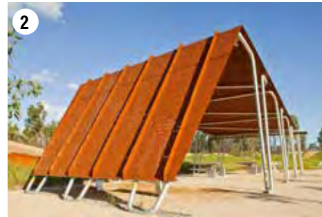
2 Trail head shelter - a basic muster point to gather and prepare before heading off to the many different trails. Wayfinding, seating and water.
