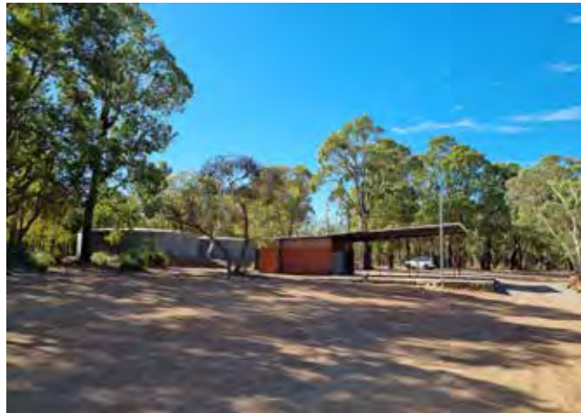
Looking north east towards the existing ablution block, DFES tanks and vehicle parking.
