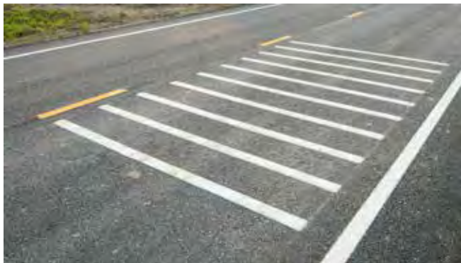
FIGURE 27. AUDIBLE ALERT FOR DRIVERS TO SLOW DOWN - RUMBLE STRIPS
