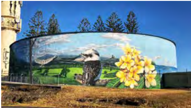
FIGURE 29. ARTWORK ON TANKS
