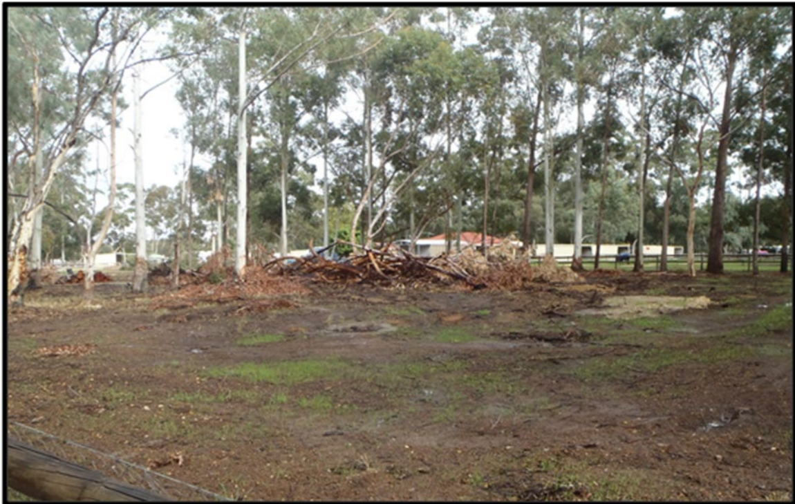
Figure 3: Removal of vegetation from site, as pictured from the north-east corner of the property
