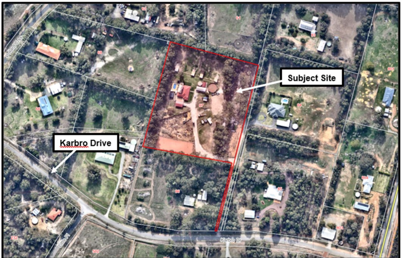
Figure 1: Aerial Imagery of the Site
