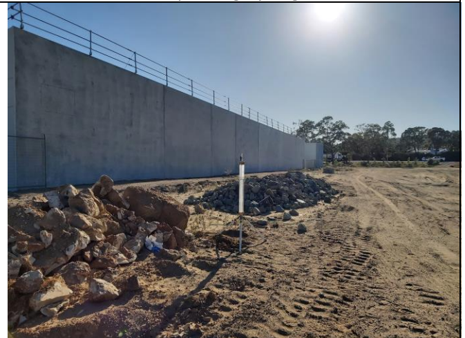
Photo 6: Conducting Field Permeability Test at FPT1
