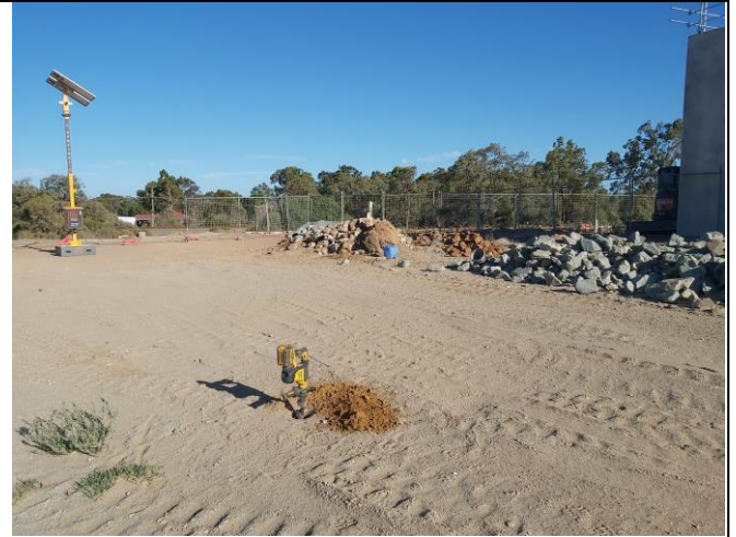
Photo 4: Subsurface probing by auger at BH1 location
