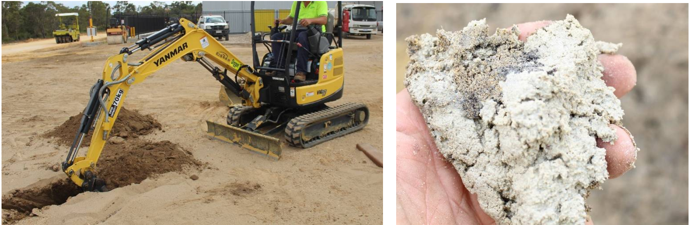
Figure 4.6 (L) Excavation of Test pit 1, showing location. (R) Moist sandy soil.
