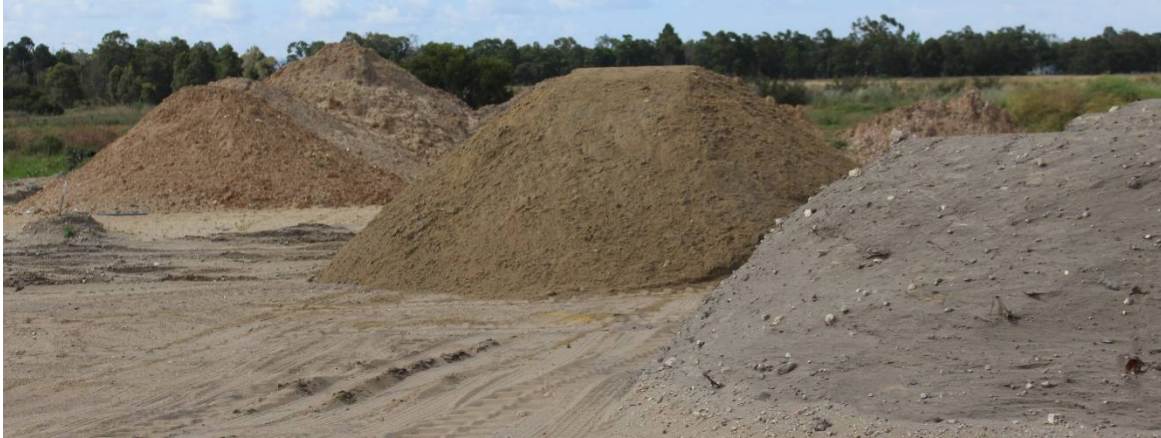
Figure 5.1 Piles of fill, typically used on site.
