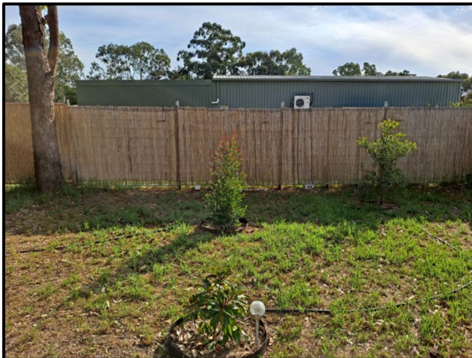
Image 2: An existing section of the fence showing the metal frame, hessian material and bamboo sheeting
