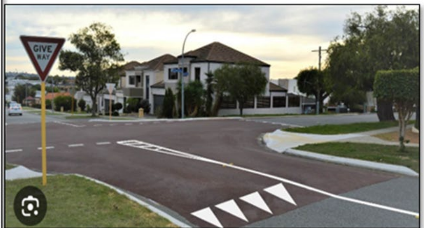
Example of Elevated Intersection
