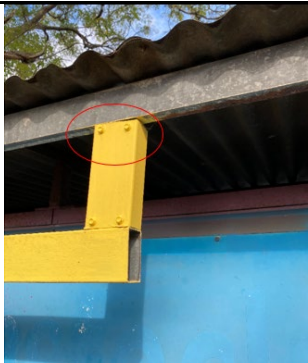
Cantilevered connection to building E
