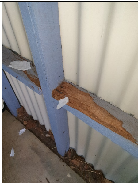
Timbers becoming flaky and powdering possibly due to termites
