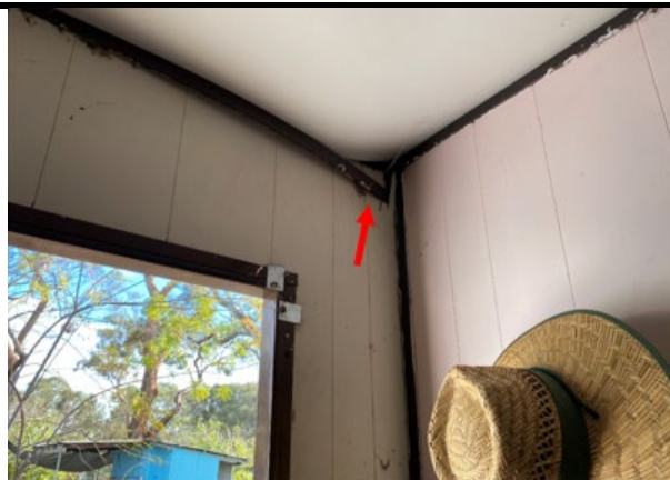
Ceiling sagging and damage
