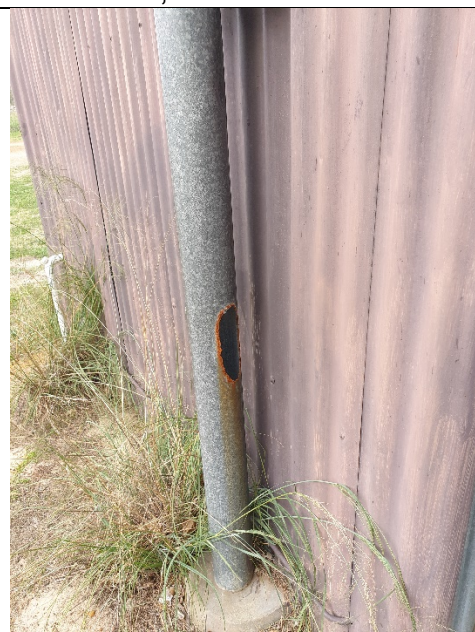
A large hole in what appears to be a ventilation stack
