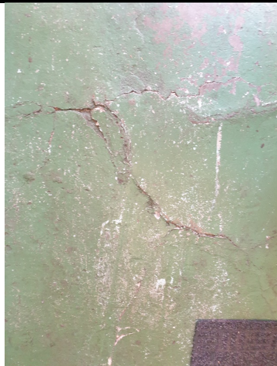
Crack in concrete slab
