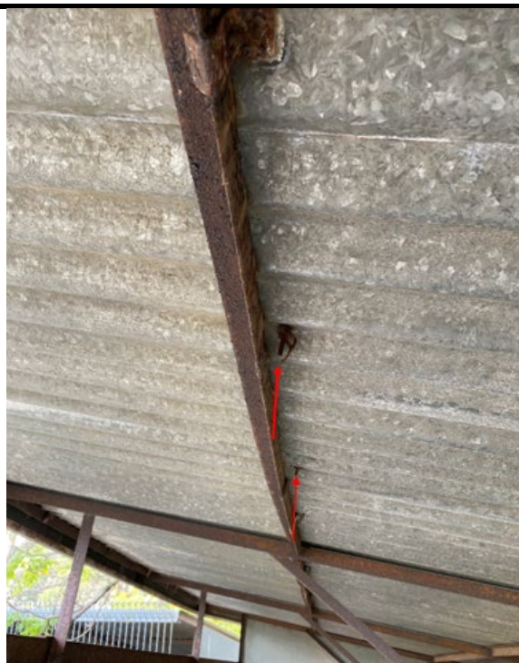
Attachment of roof sheeting corroded
