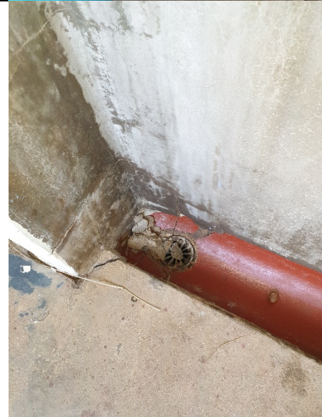
Concrete in urinal deteriorating and cracking causing debris in drain
