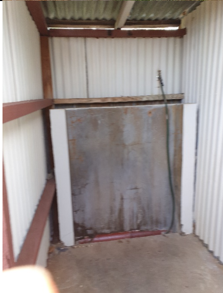
Concrete wall type urinal with hose attachment as flush
