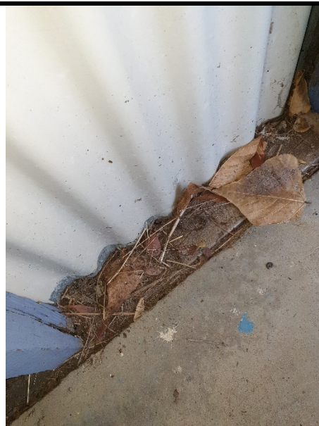
Timbers at base of frame with possible wet rot
