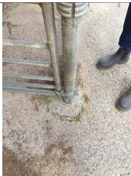
It appears new posts have been installed with new footings
