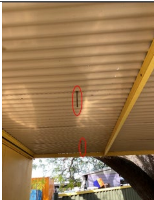
Bolts from roof used to hold up server door
