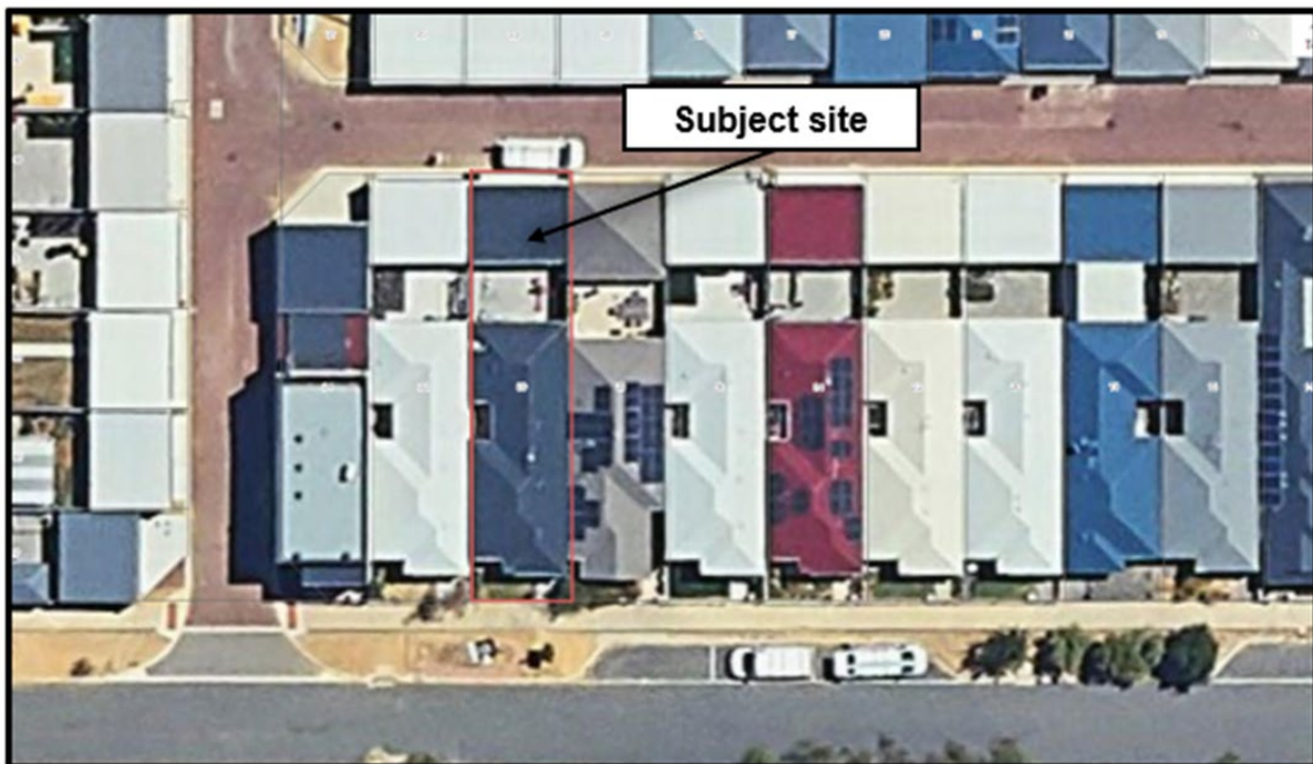
Image 1 - Aerial of subject site
