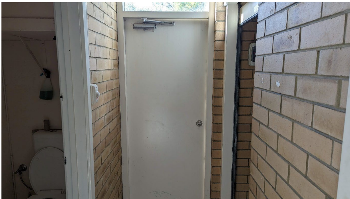
External access to toilets for general public
