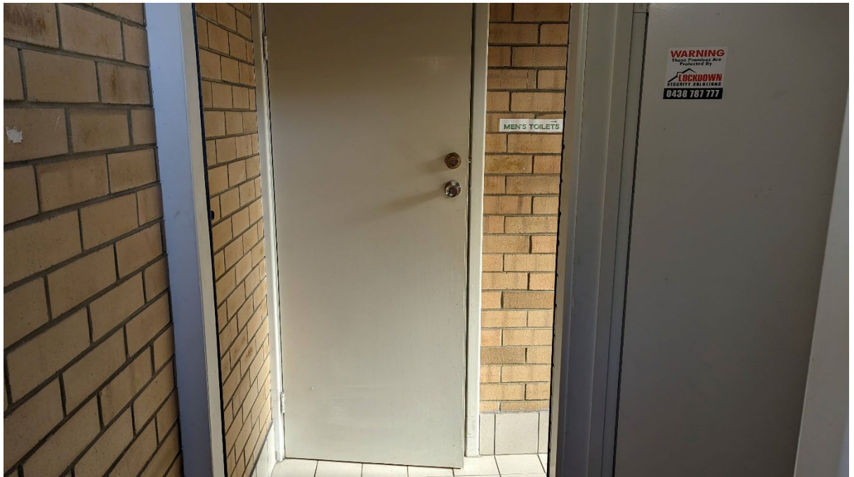
Entry to Men's Toilets
