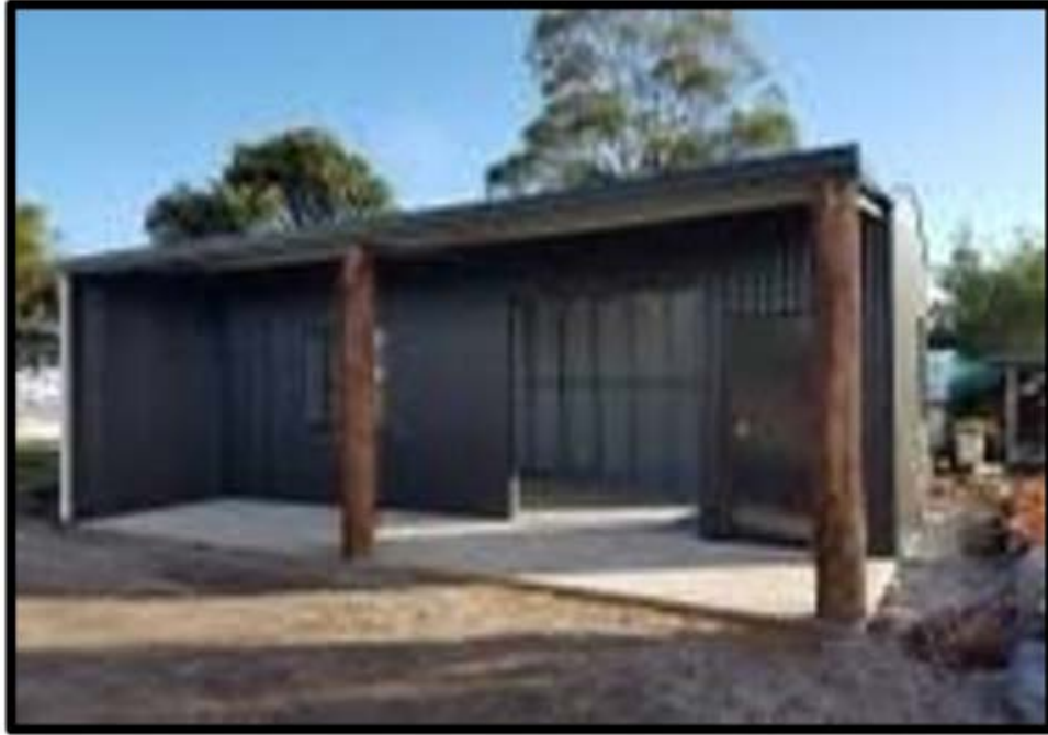
Figure 4 – Illustration of outbuilding incorporating bush poles
