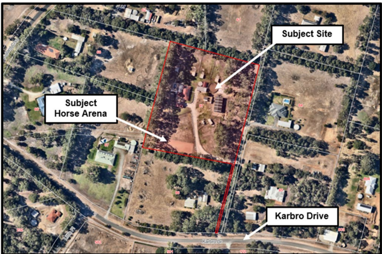
Figure 1: Aerial imagery of the site
