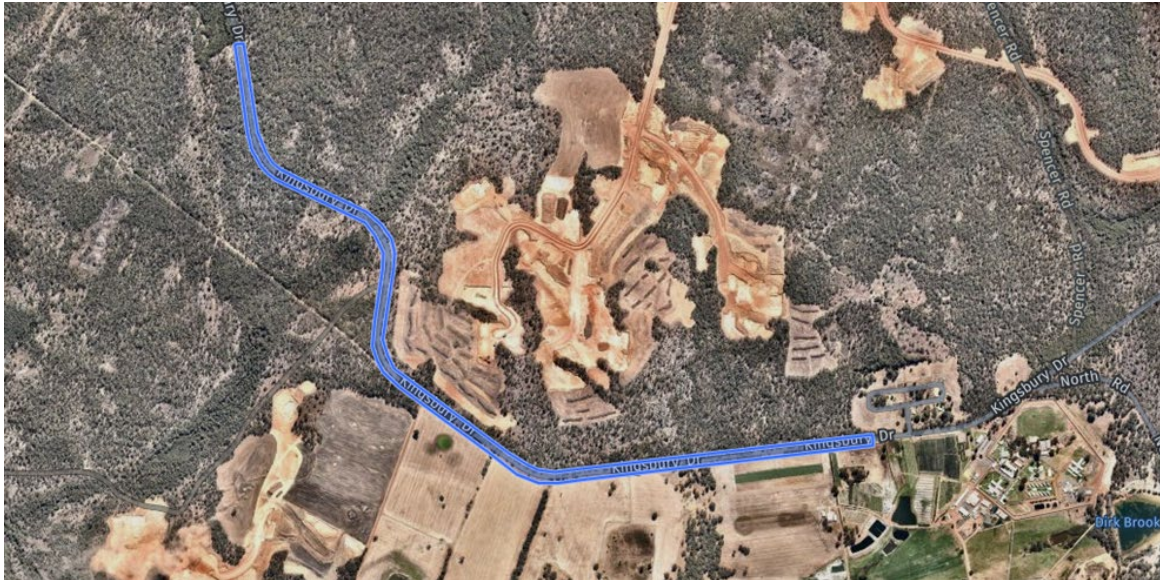
Figure 1: Aerial view – Kingsbury Drive SLK 7.0 to SLK 9.1
