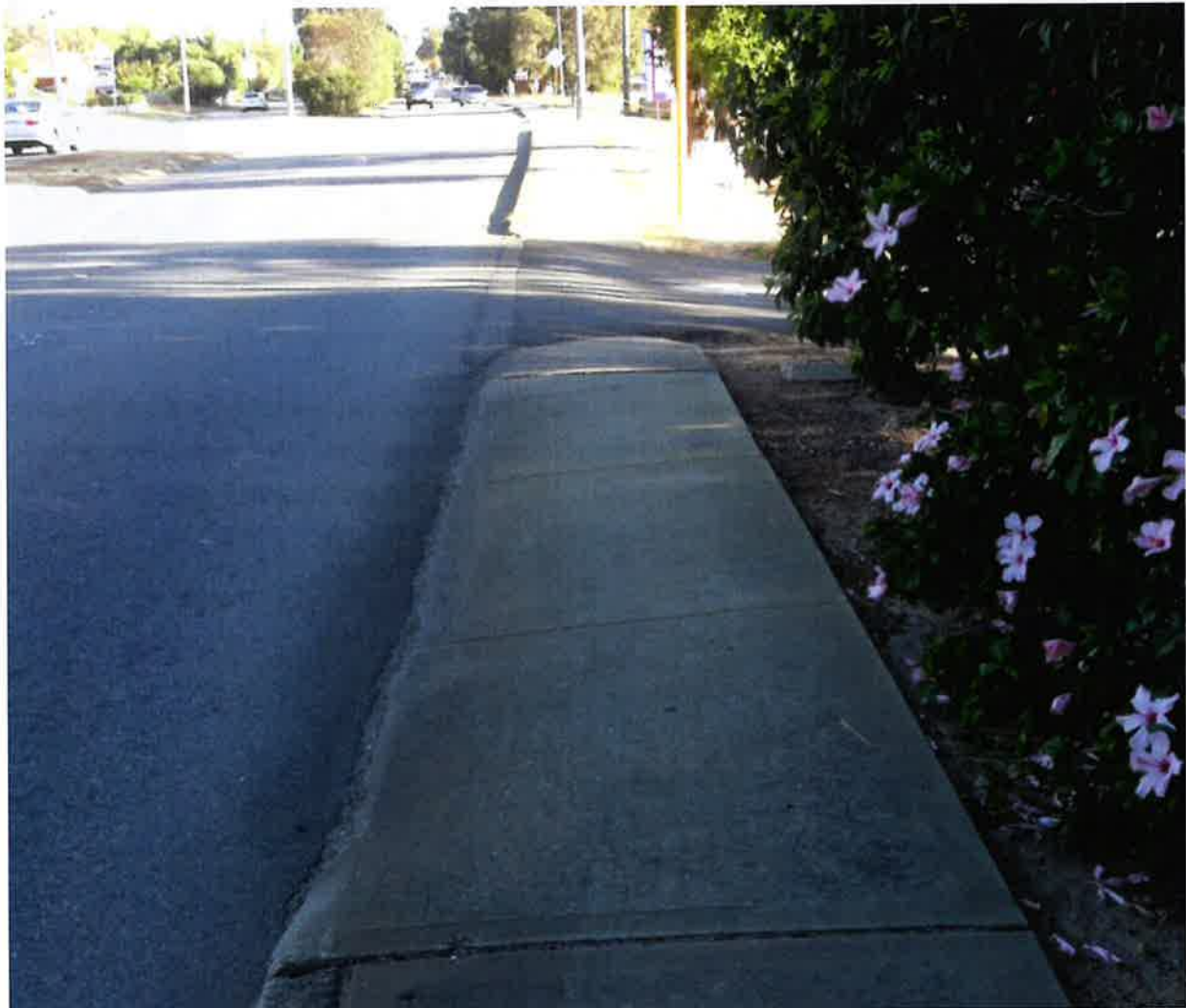
Photograph 15 – Example of South Western Hwy path on west side sloping towards traffic
