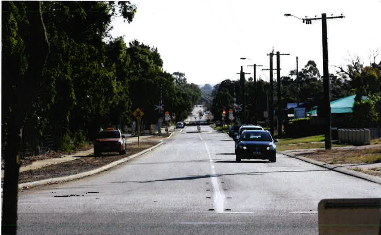
Photograph 5 – Looking west on Larsen Rd from South Western Hwy (subject site on left)
