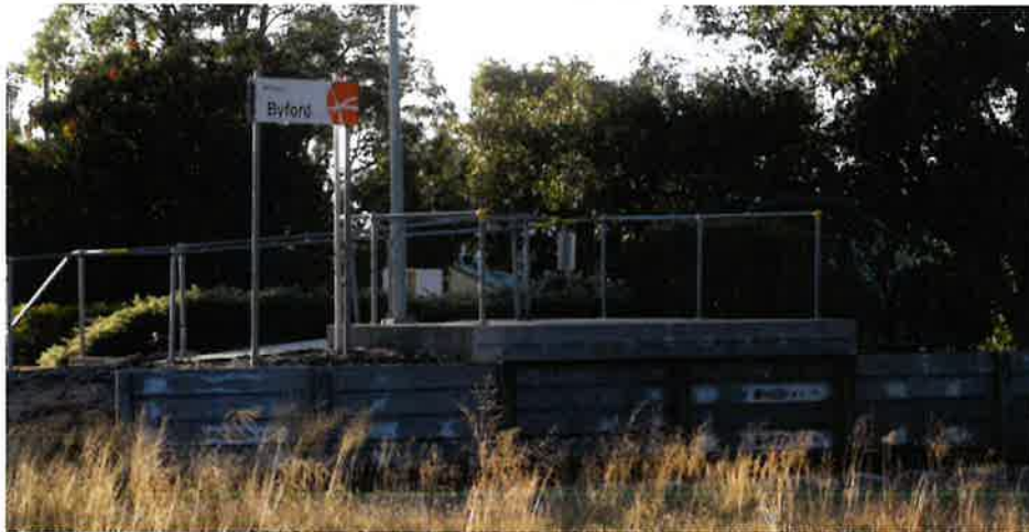
Photograph 14 – Existing Byford train station
