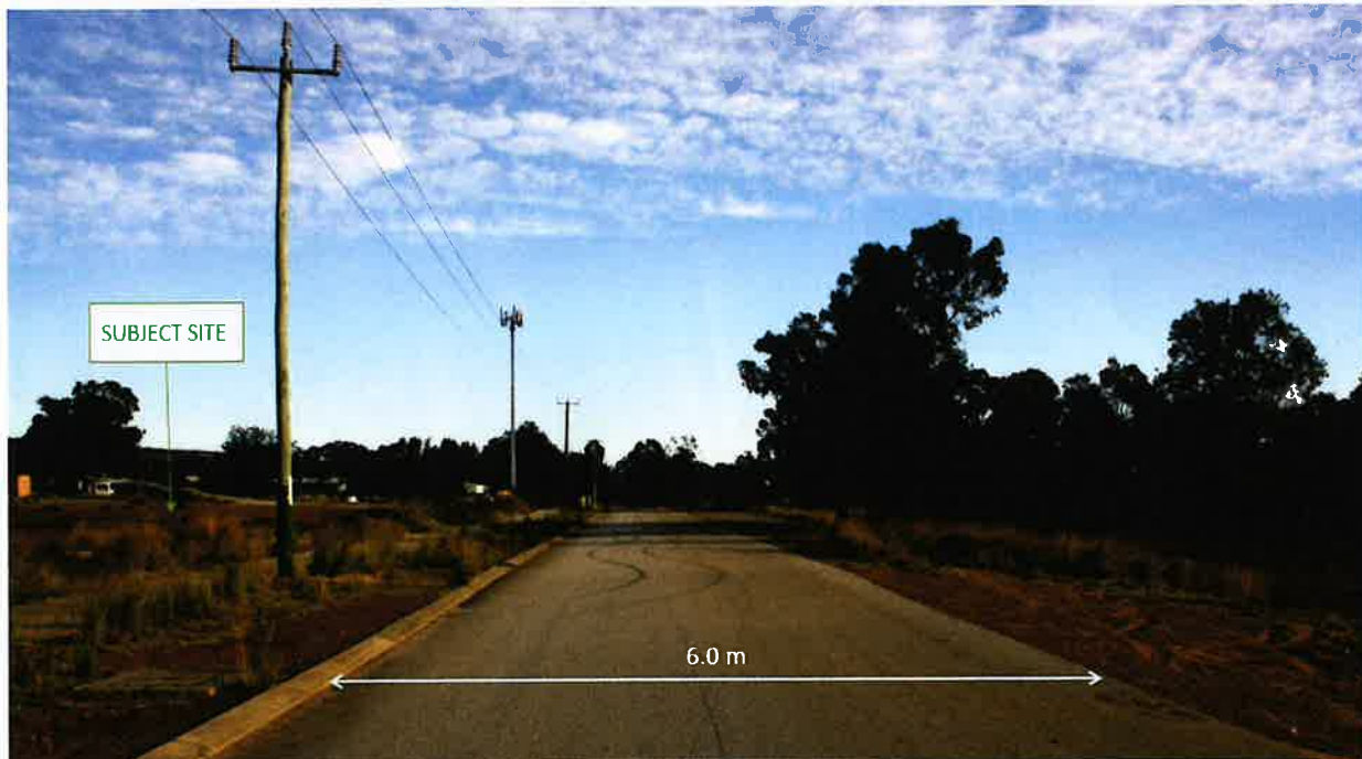
Photograph 7 – Typical cross section of George St
