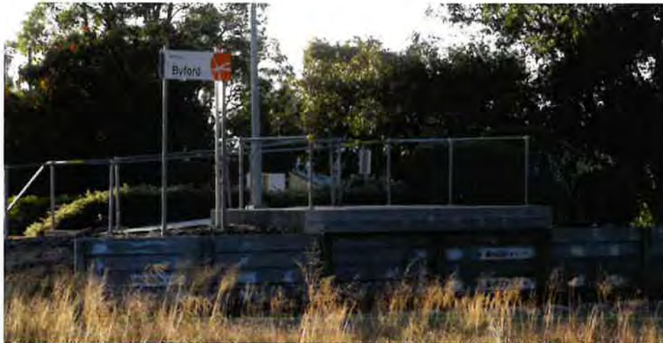
Photograph 14 – Existing Byford train station
