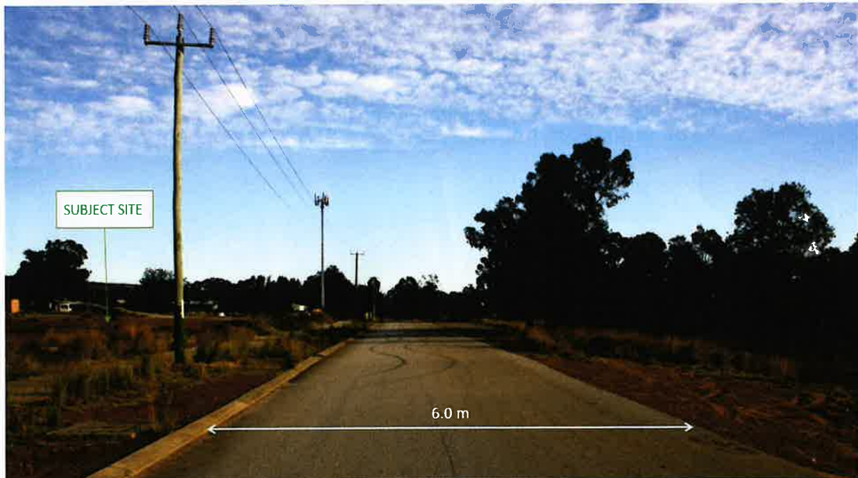
Photograph 7 – Typical cross section of George St
