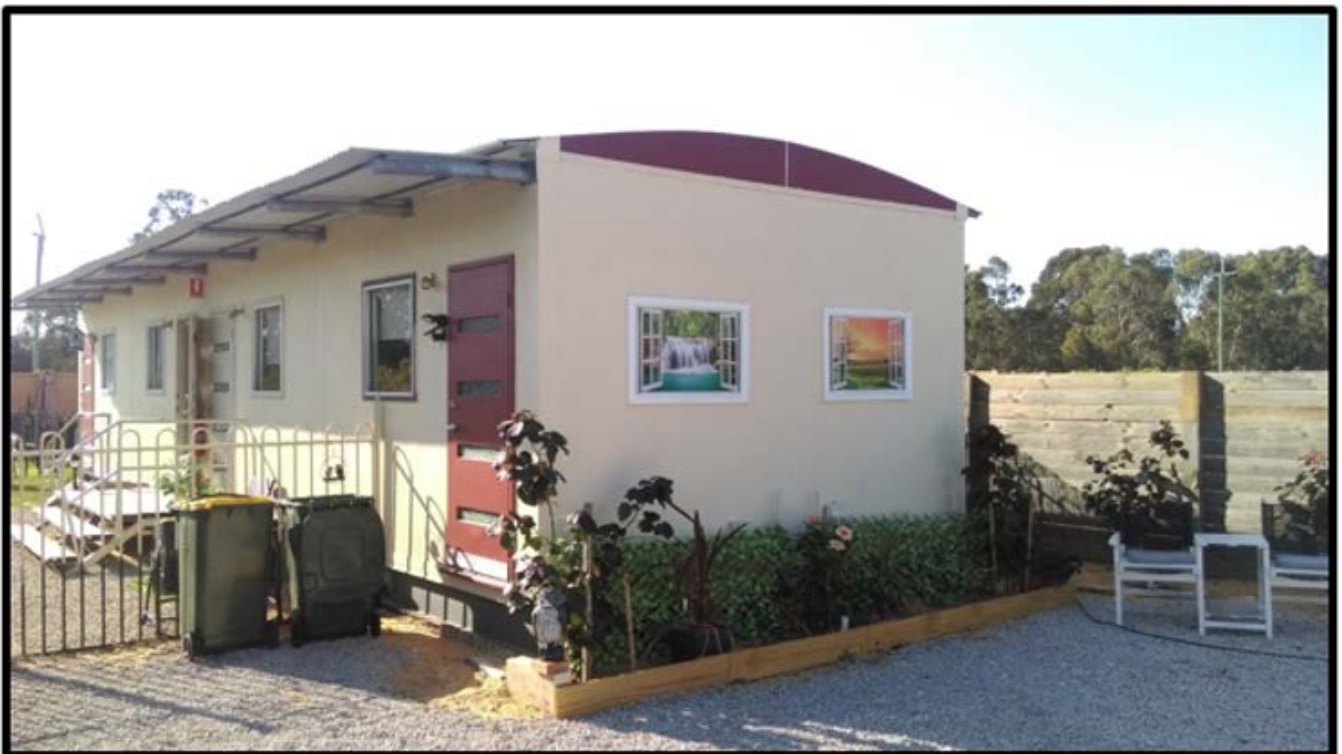
Figure 5: The existing temporary accommodation
