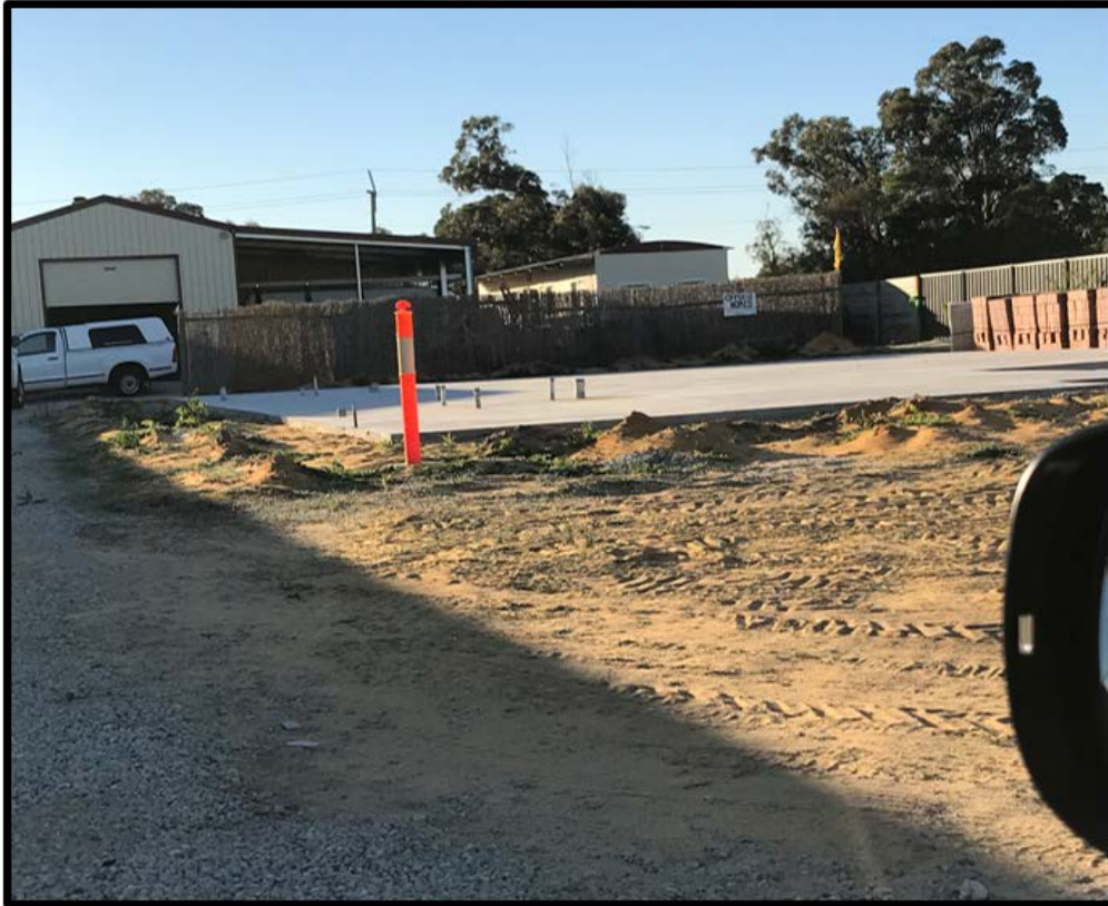
Figure 3: Subject site and the dwelling June 2019
