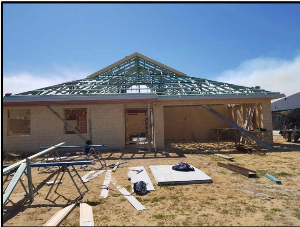
Figure 4: Subject site and the dwelling September 2020
