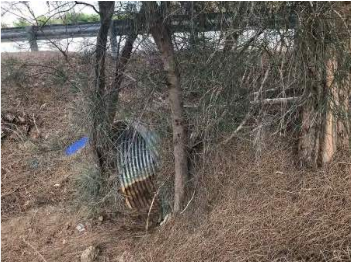
Structure No 19: Site 1.5 – Thomas Road, Ballak Place Intersection
