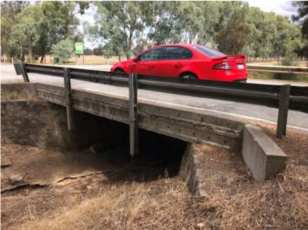
Structure No 81: Site 1.7 – Birrega Subdrain at Abernethy Road, Kargotich Road Intersection
