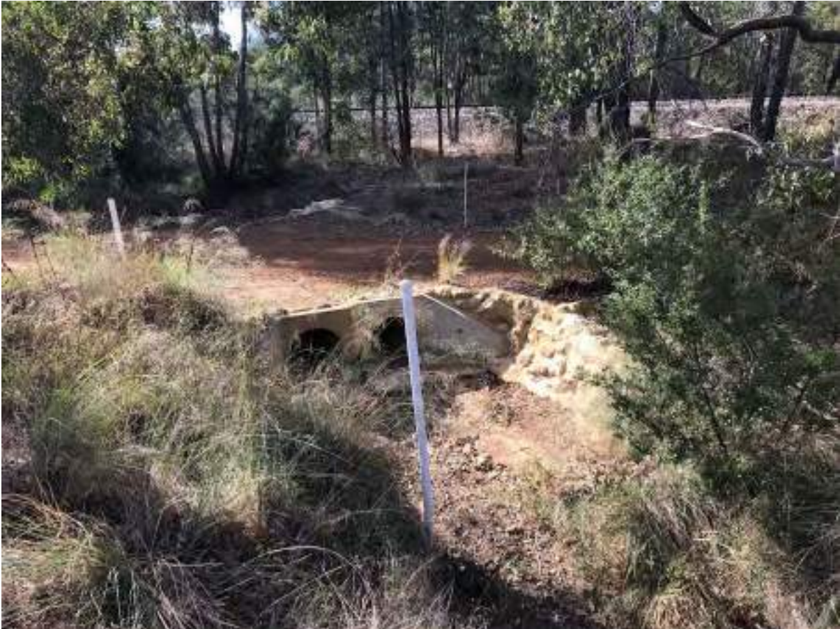
Structure No 94: Site 2.8 – Norman Drain at Railway walk trail
