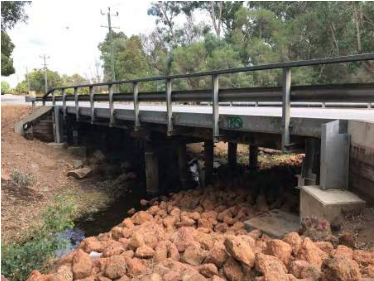
Structure No 3: Site 1.23 – Wungong River at Rowley Road
