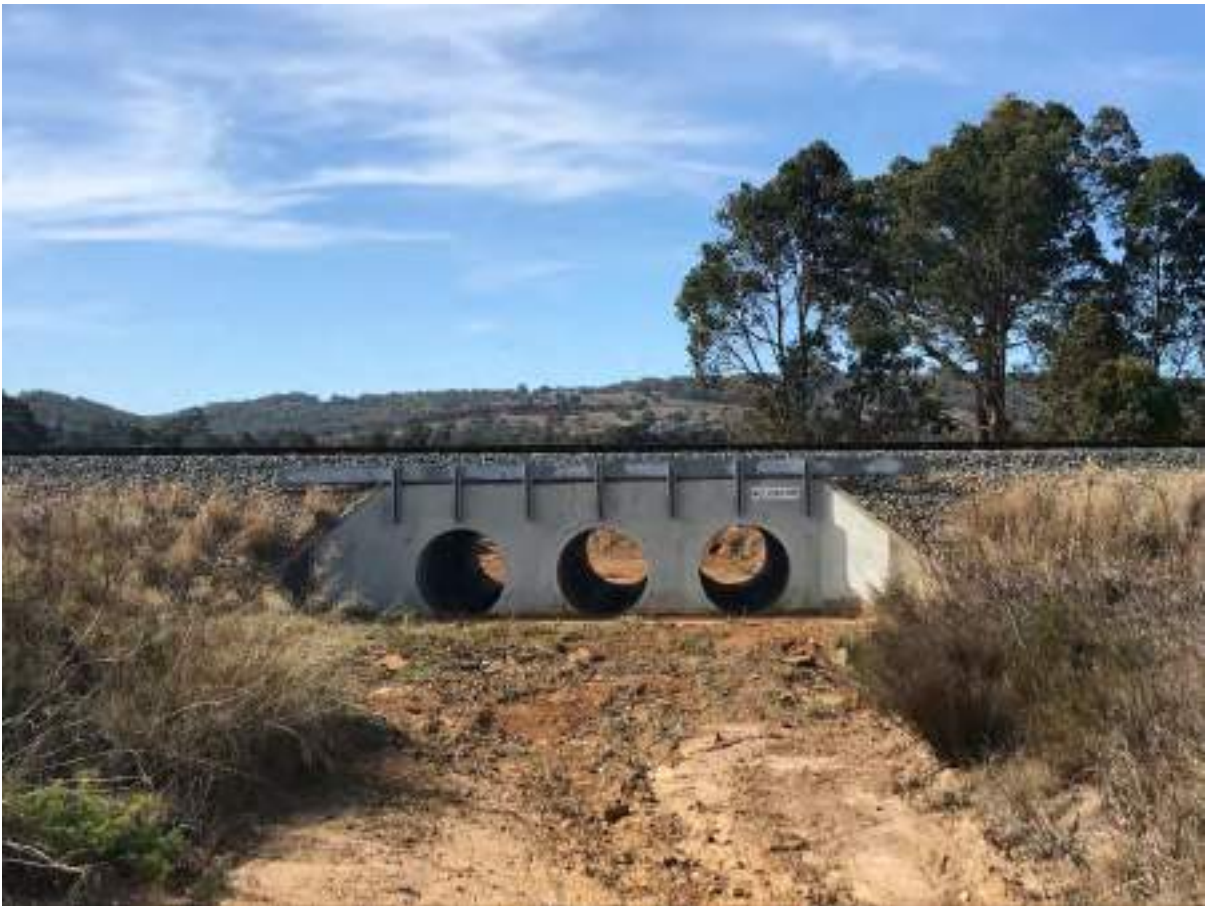
Structure No 86: Site 2.10 – Cardup Drain at Railway
