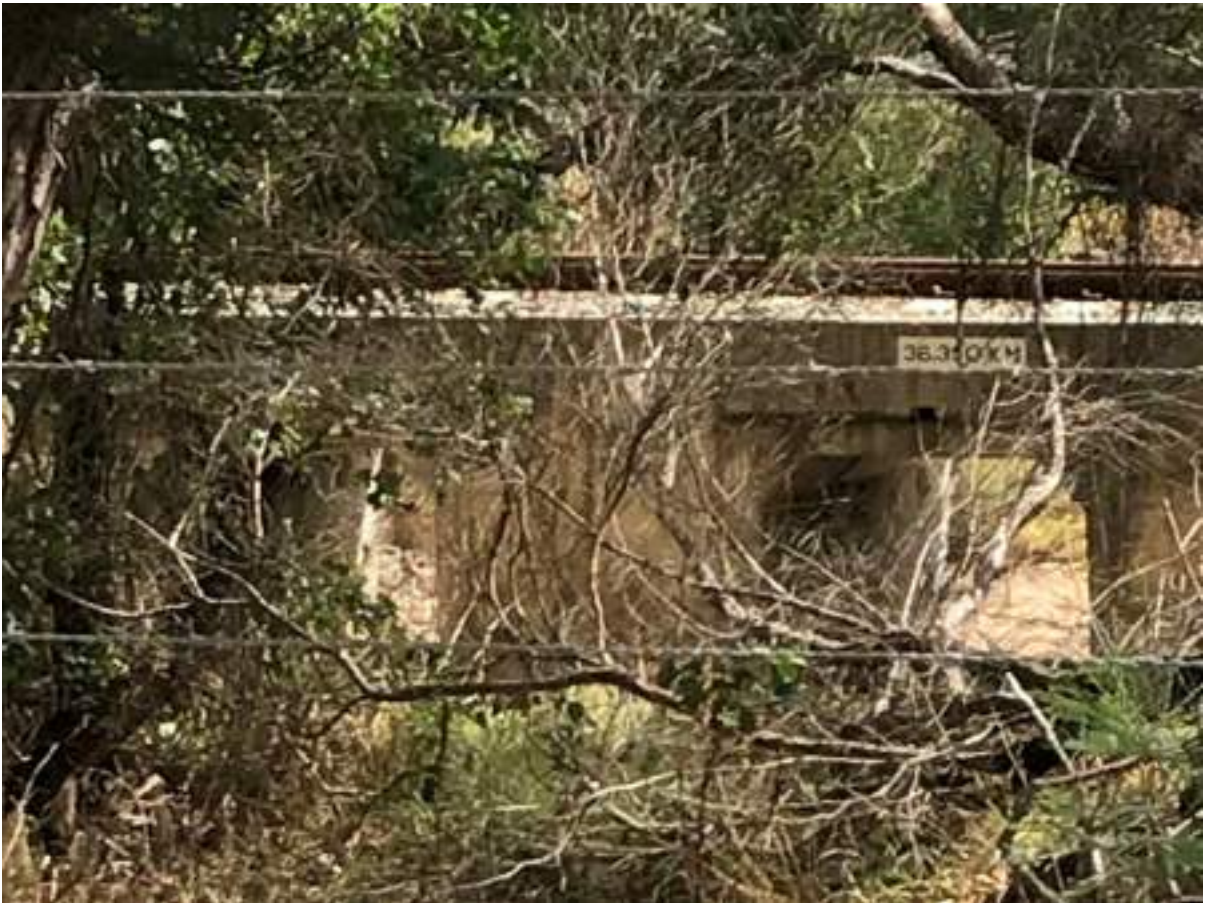
Structure No 31: Site 1.15 – Oaklands Drain at Railway
