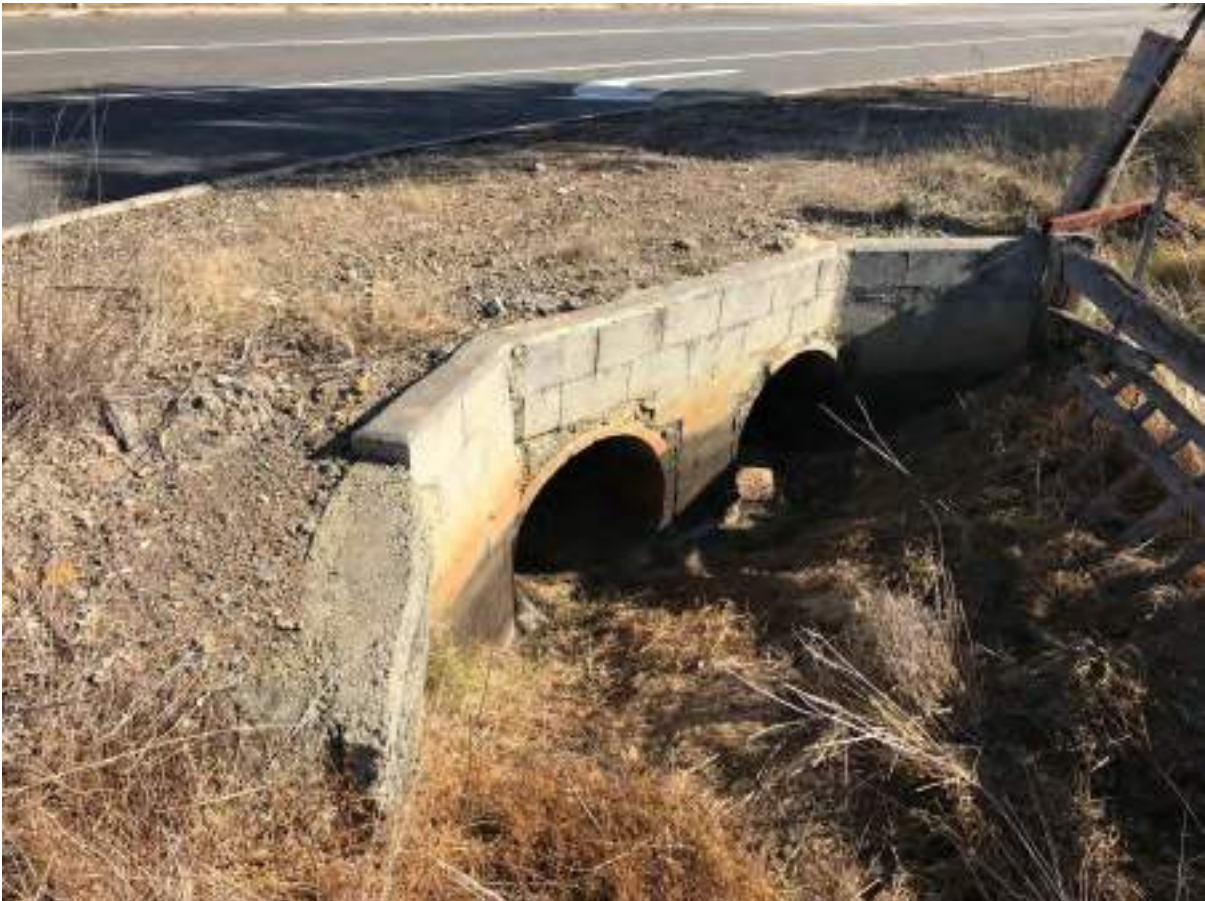
Structure No 98: Site 2.5 – Norman Drain at Kargotich Road
