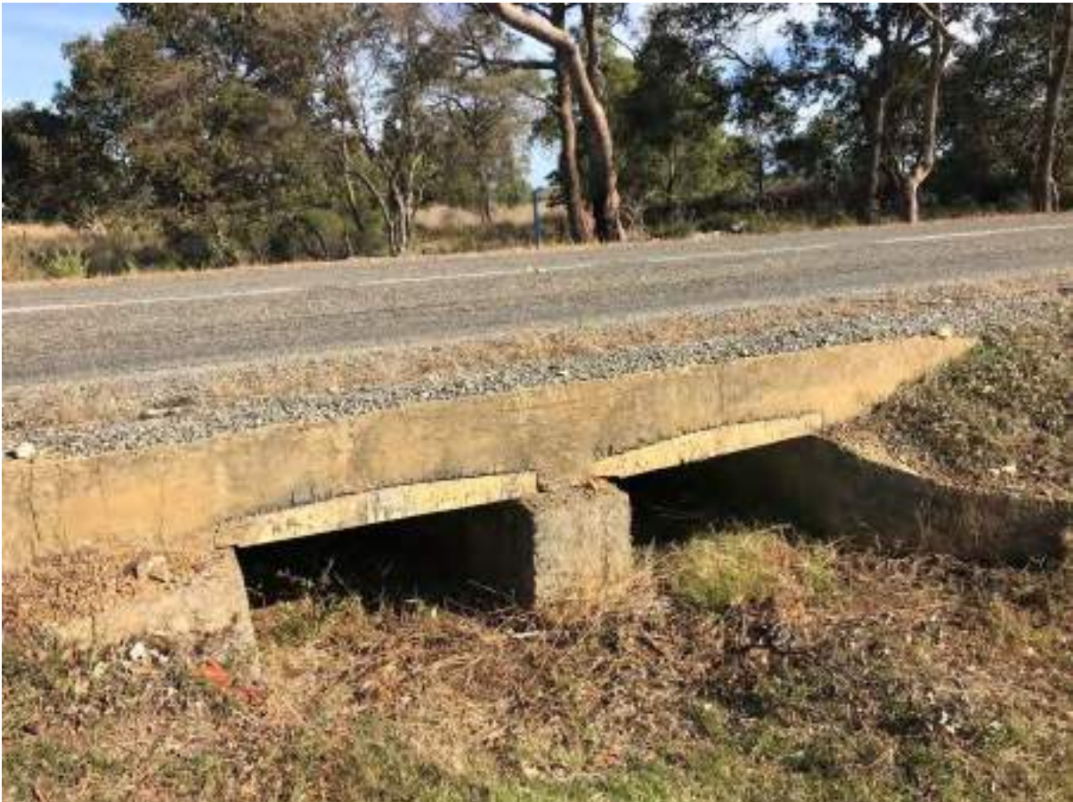
Structure No 91: Site 2.14 – Cardup Drain at Hopkinson Road
