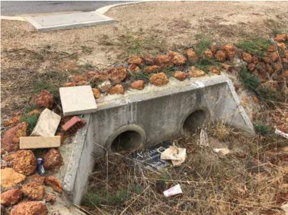
Structure No 50: Site 1.24 – Beenyup Brook Subdrain at Abernethy Road
