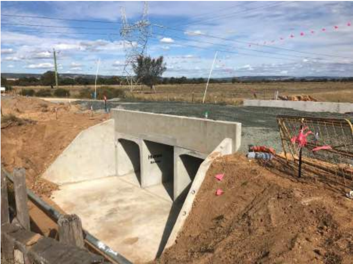
Structure No 54: Site 1.10 – Oaklands Drain at Gossage Road
