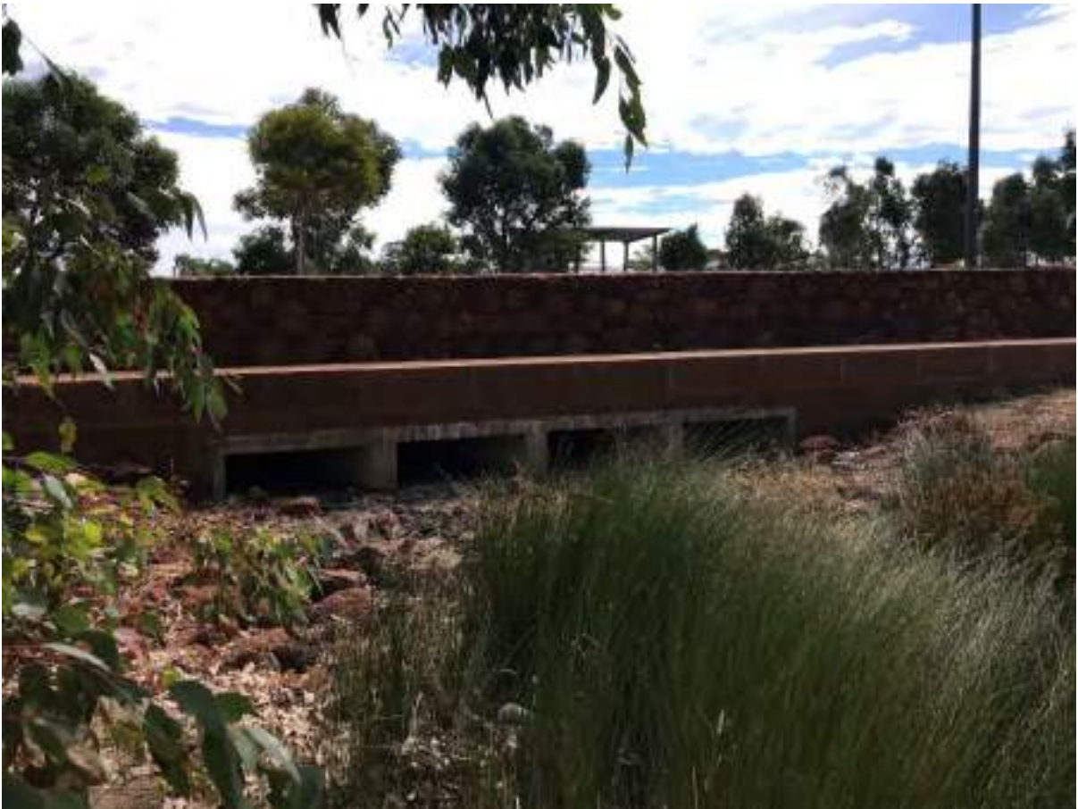
Structure No 60: Site 1.20 – Glades Multiple Use Corridor at Doley Road
