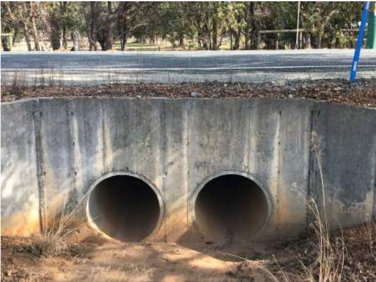
Structure No 88: Site 2.10 – Cardup Drain at Soldiers Road
