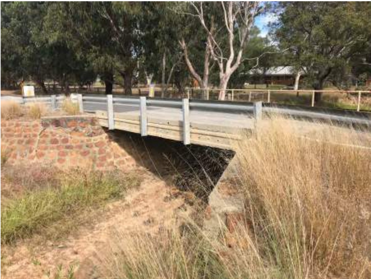
Structure No 82: Site 1.11 – Birrega Subdrain at Orton Road, Kargotich Road Intersection
