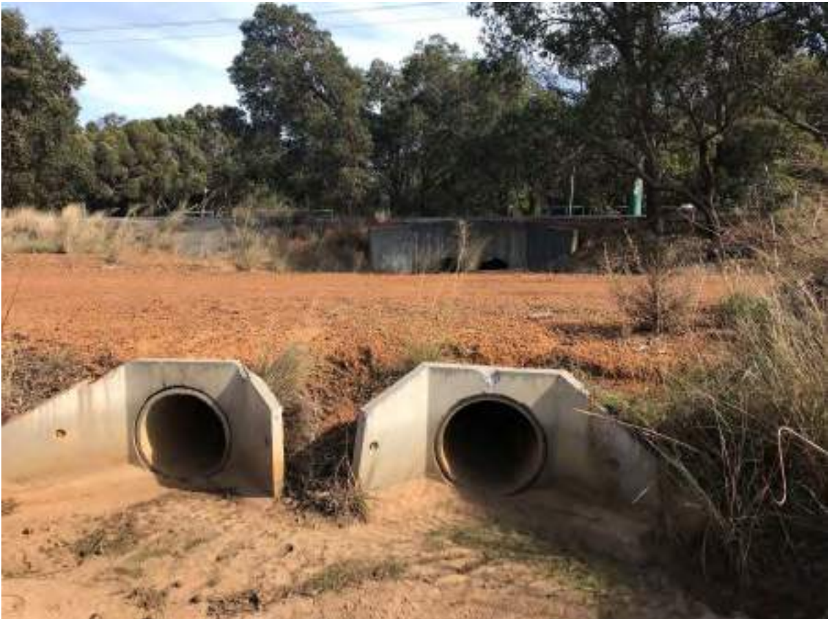
Structure No 87: Site 2.10 – Cardup Drain at Railway walk trail
