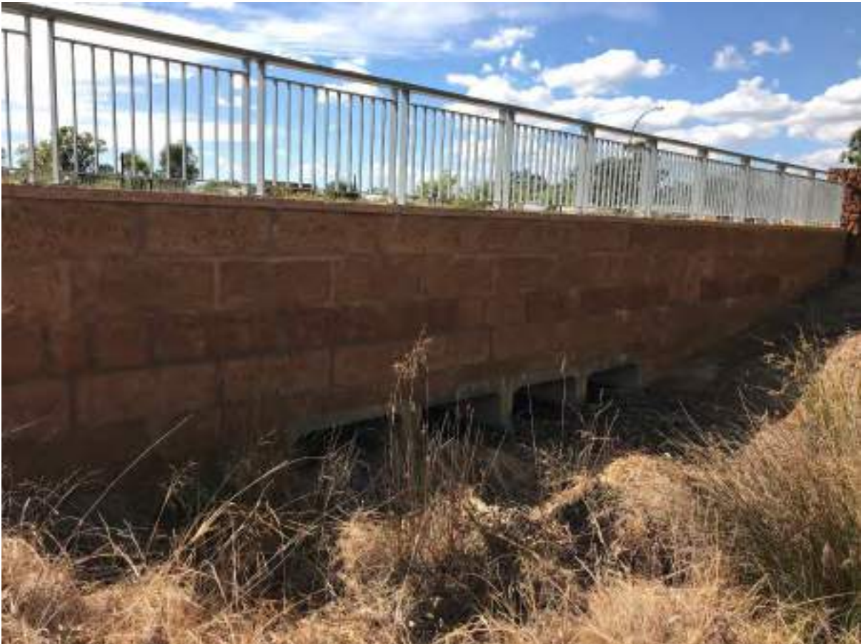
Structure No 58: Site 1.20 – Glades Multiple Use Corridor at Mead Street
