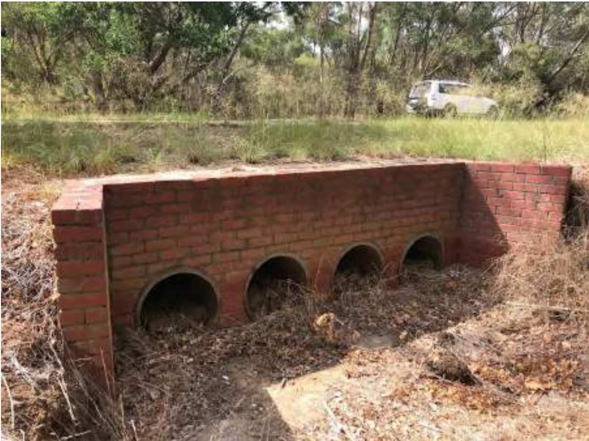
Structure No 6: Site 1.22 – Birrega Drain at Wungong South Road
