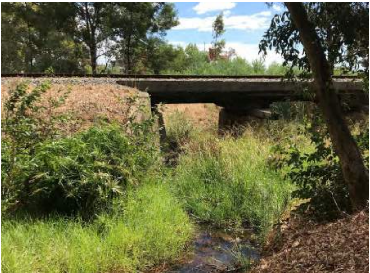
Structure No 40: Site 1.2 – Beenyup Brook at Railway
