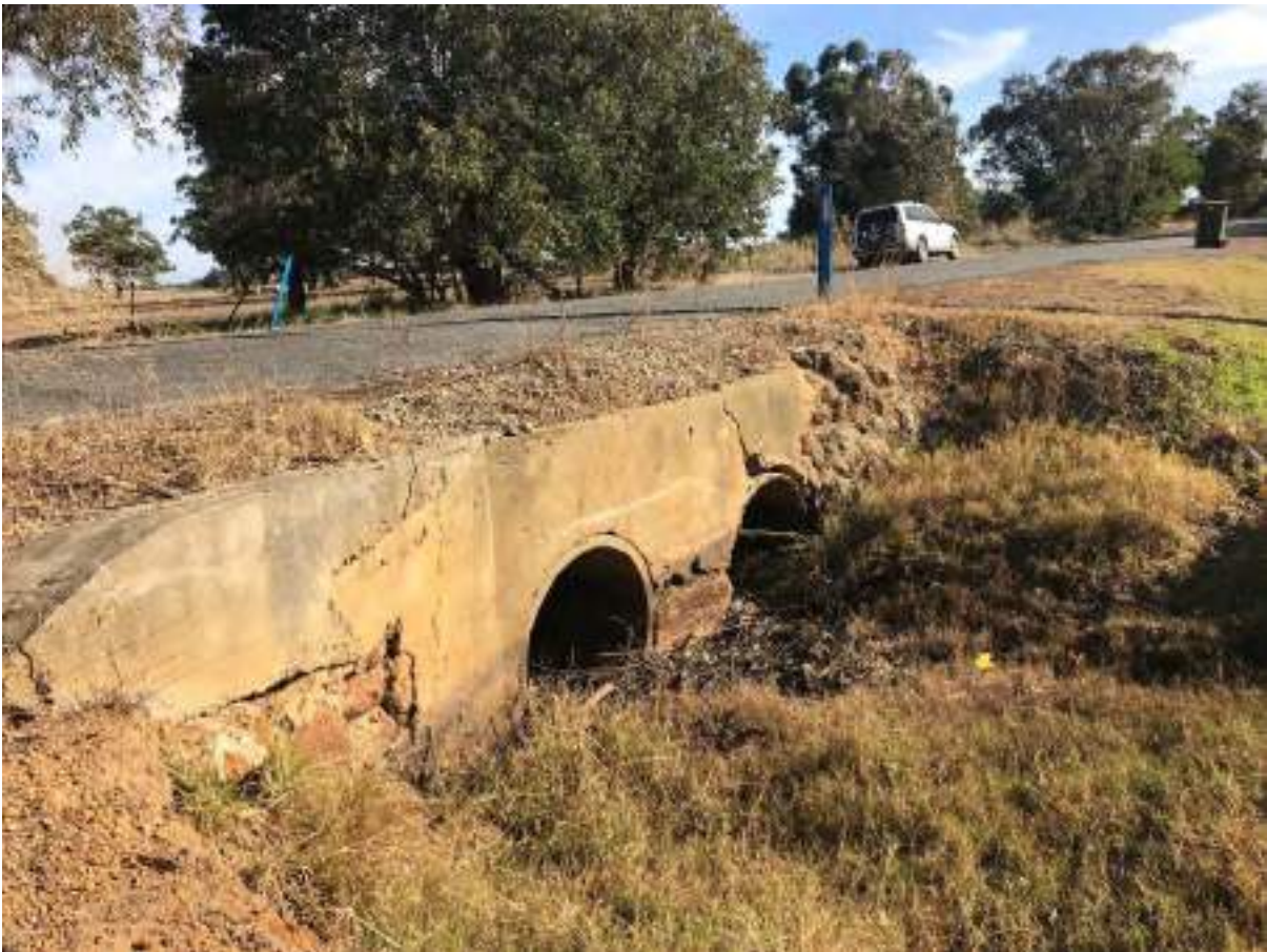
Structure No 96: Site 2.7 – Norman Drain at Hopkinson Road
