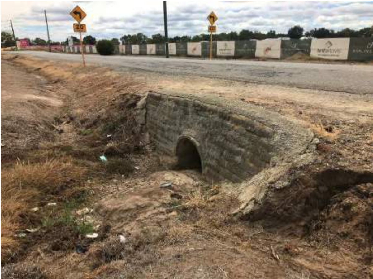
Structure No 8: Site 1.1 – Hopkinson Road at Darling Downs
