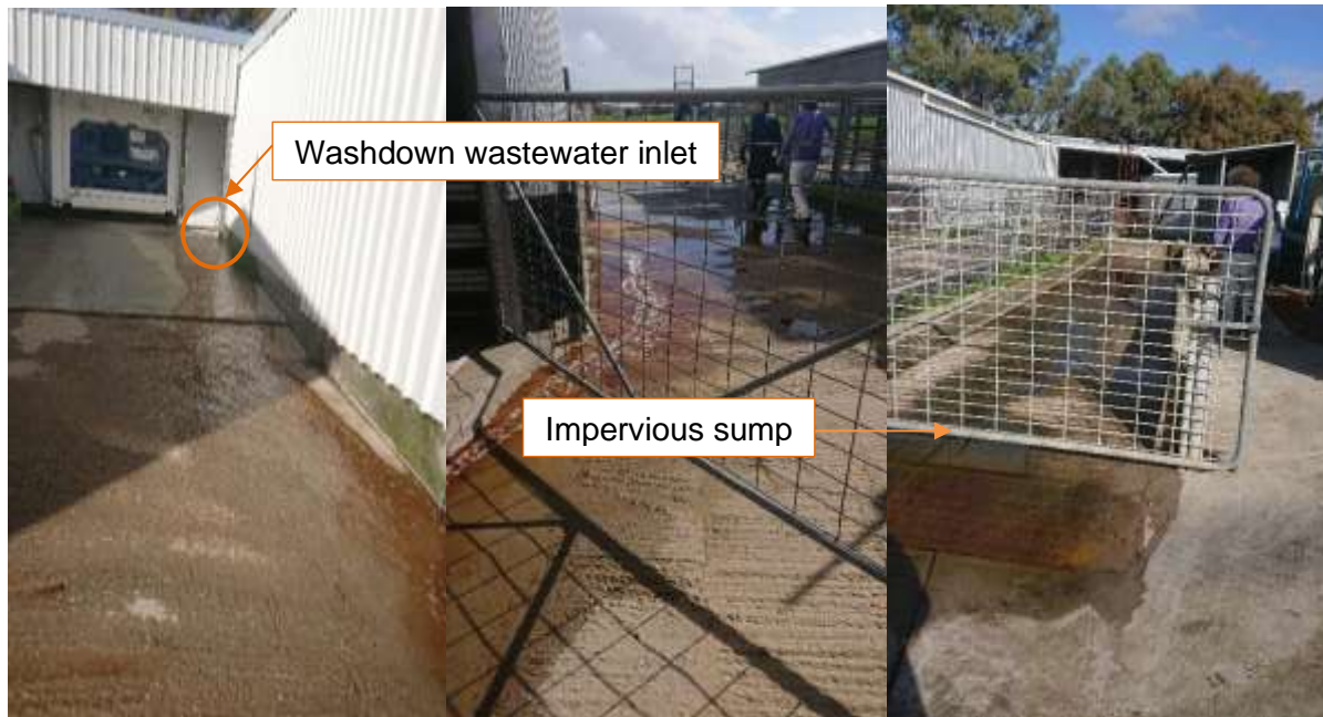
Plates 4: Concrete sump
