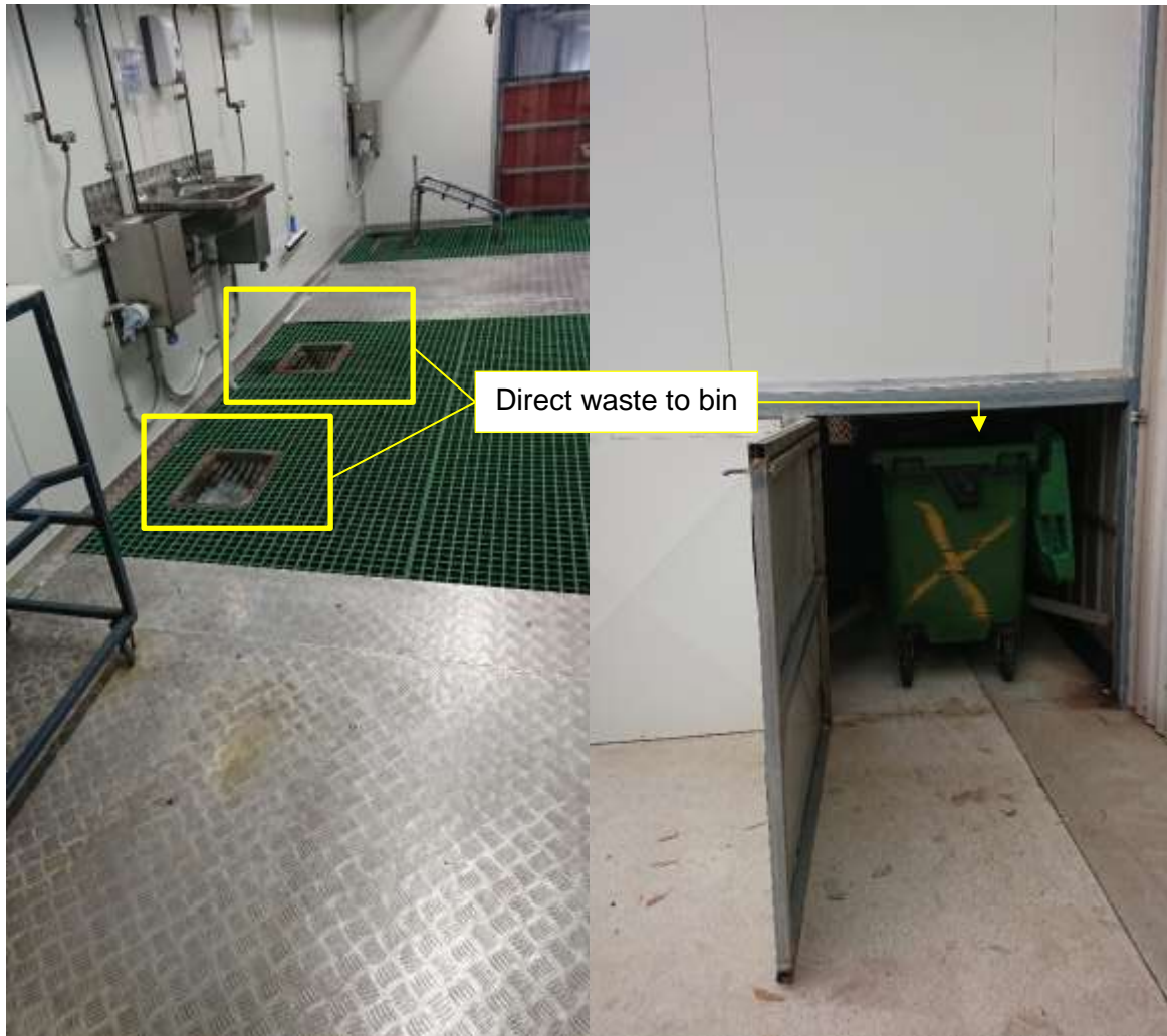
Plates 2: Bin beneath floor
