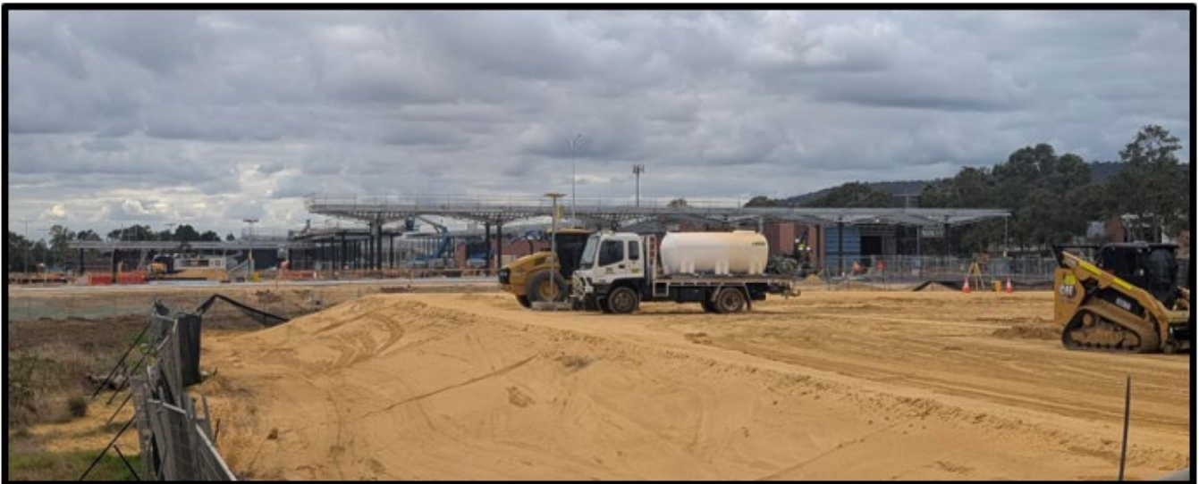
Figure 3 - The Future Byford Railway Station
