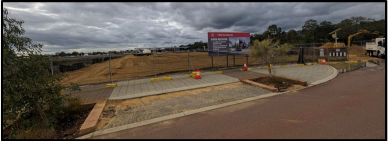
Figure 2 - Current Site Photographs
