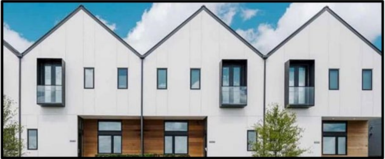
Figure 19 - Design features, including recessed walls, balconies and interesting design features
