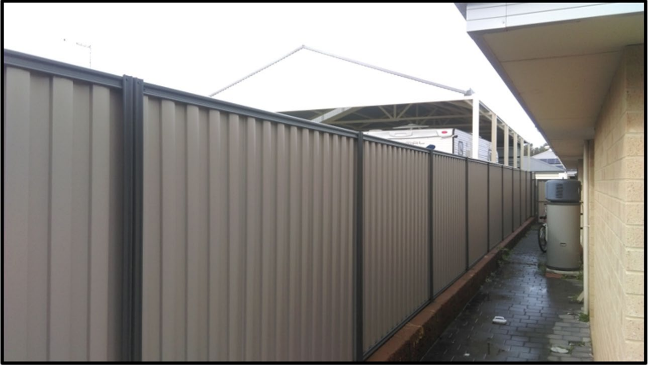
Figure 6: Proposed development location to the rear of the existing carport as viewed from the rear of the neighbouring block
