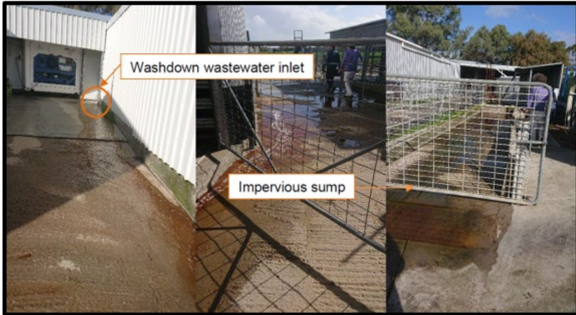
Figure 5: Wastewater exits the processing area and gathers in the sump
