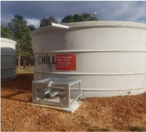
Strategic 47,000 Litre Concrete Tank & Protected Fittings
