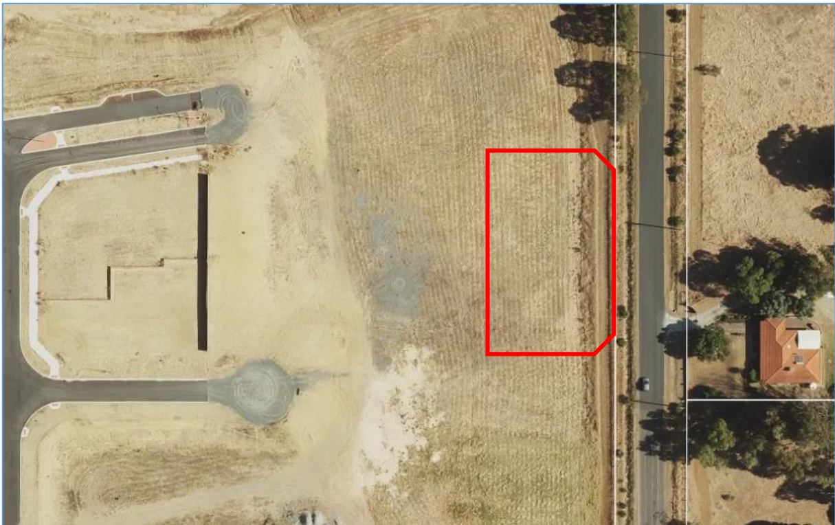
Figure 2: Aerial View (December 2022)
