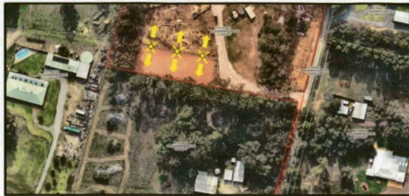
Figure 9: Existing arena light position angled towards neighbouring properties
