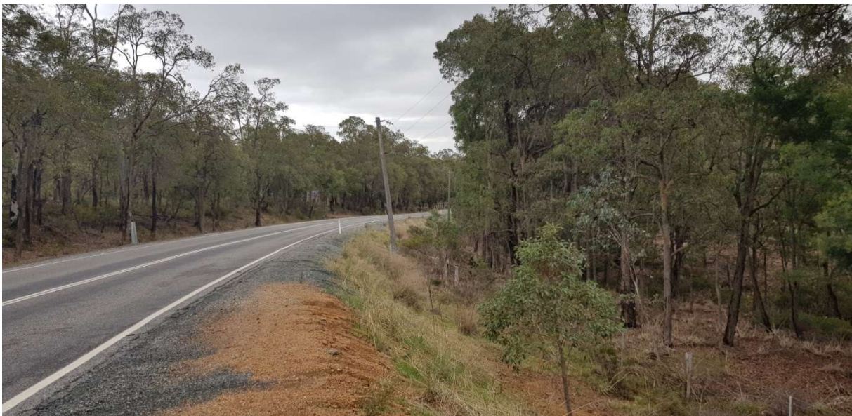
Figure 3: Finding 2.1 - Steep Batter Slopes
