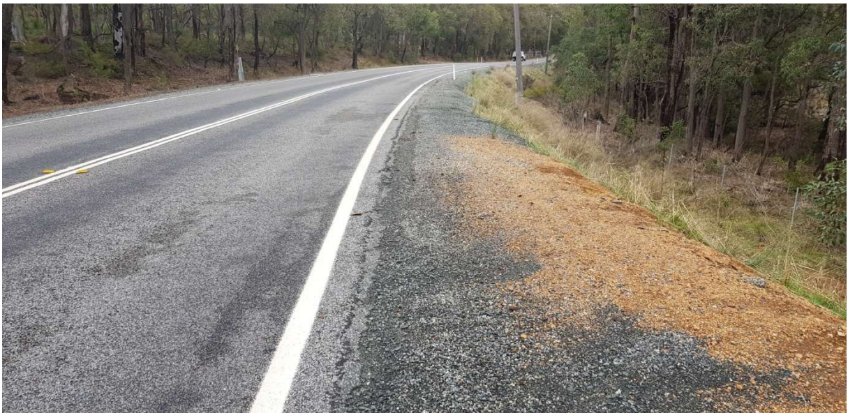
Figure 6: Finding 2.4 Unsealed Shoulder
