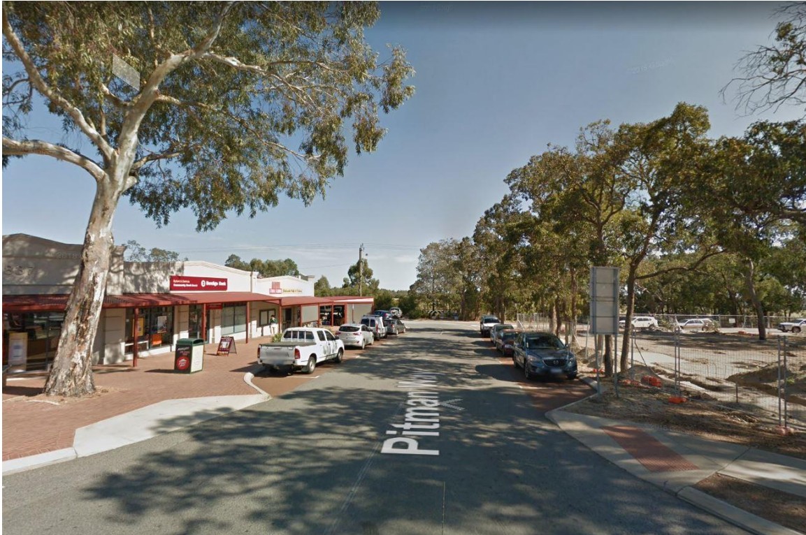
Figure 10. Westbound view along Pitman
