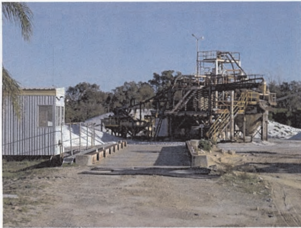
Existing weighbridge and wash plant
