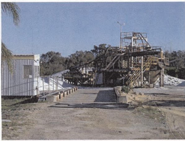
Existing weighbridge and wash plant
