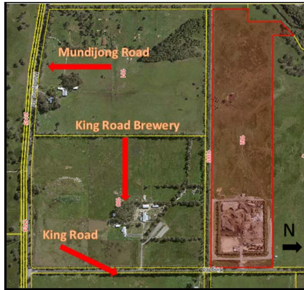
Figure 1: Aerial of site in relation to King Road and Mundijong Road
