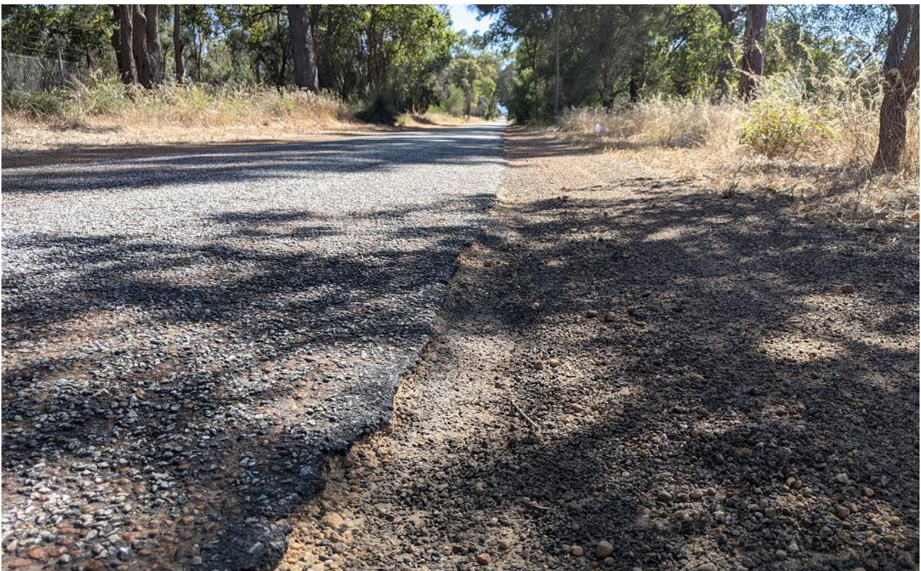
Figure 2-1 Damaged Carriageway
