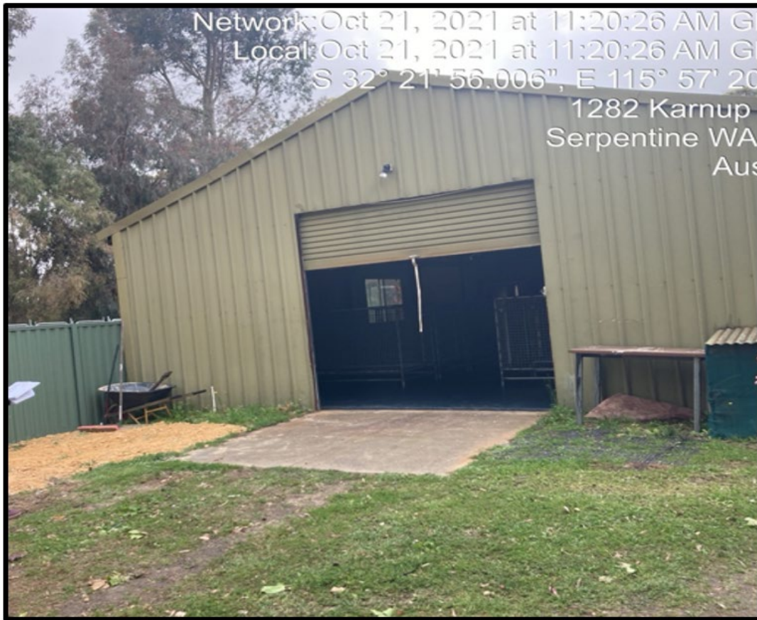
Figure 4: Existing shed with Kennels
