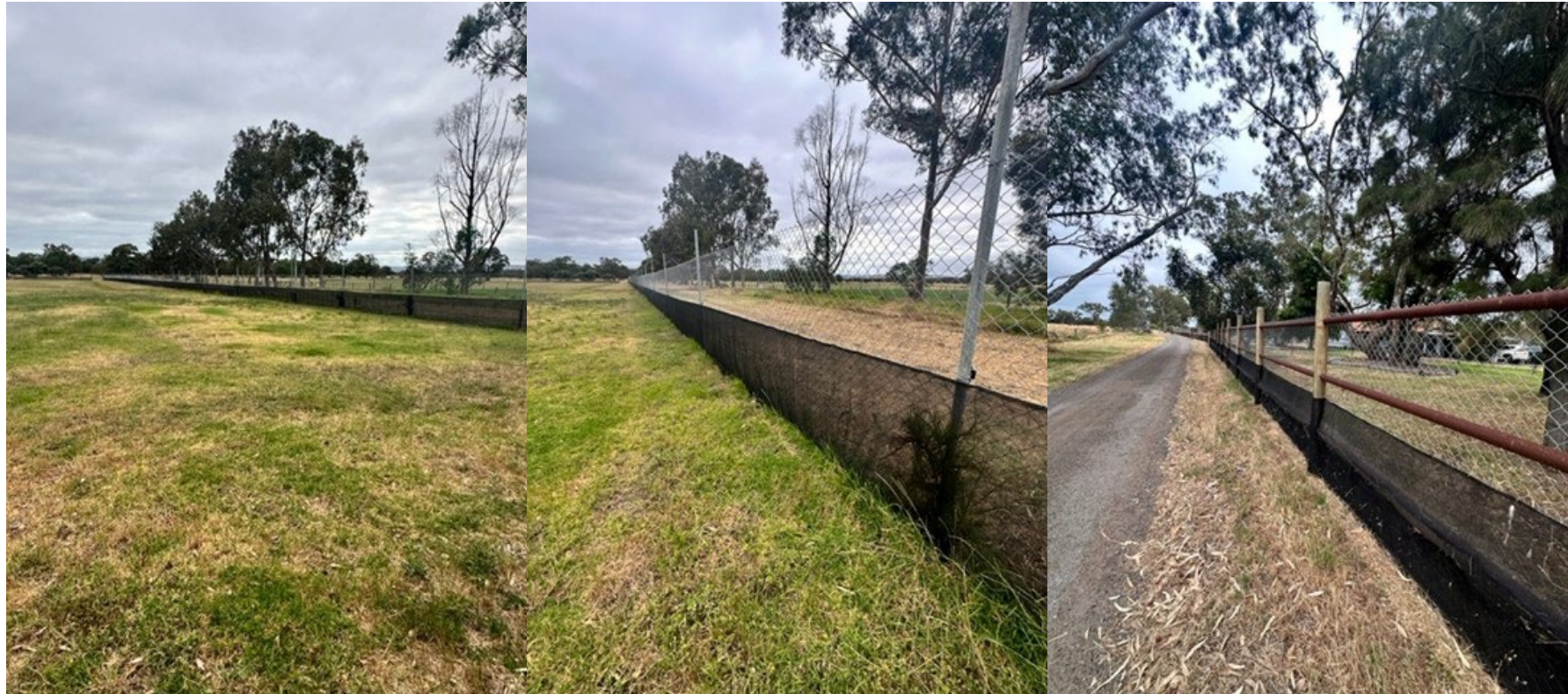
Dog Boundary Fences Photo 1 & 2 is the boundary to the North, South, and East. Photo 3 is the boundary to the West
