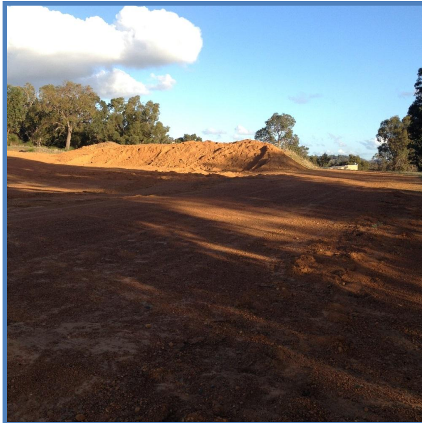
Location of proposed shed looking south (adjoining property outbuilding is visible)
