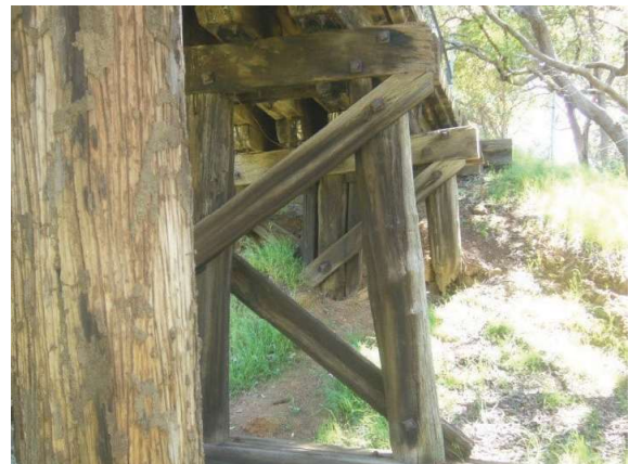
Brickworks Railway Bridge, view looking North Source: Stephen Carrick Architects 2014 (SJ1-01 pic 5)
