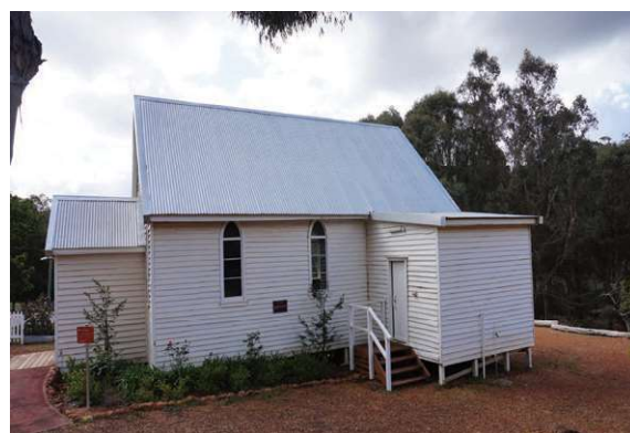
Side View, East
