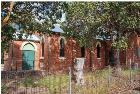
Side elevation, looking south east
