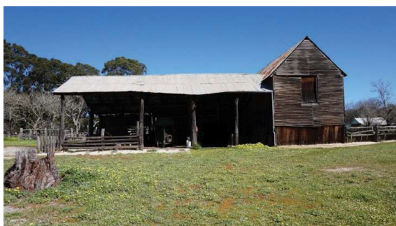
Thomas Peel's Barn c1840 (North looking South view)
