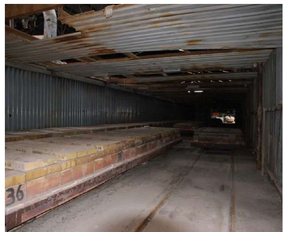
Dryer view northern side
