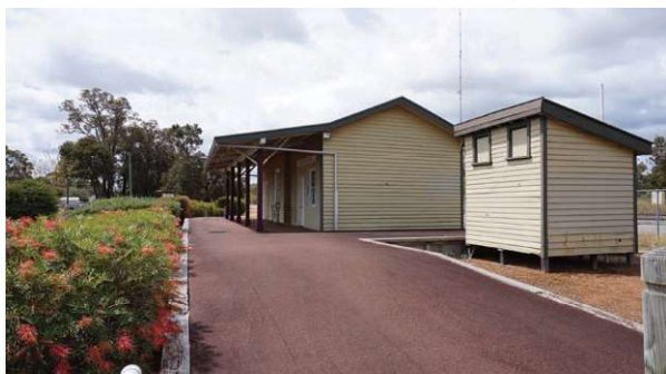
View North along platform
