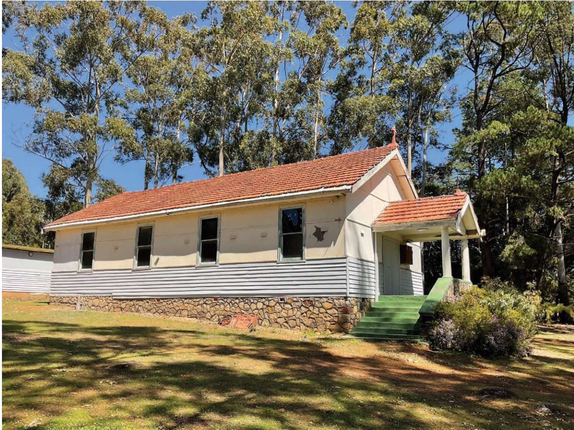
St. Maria Goretti Church – East Side View – Source: Stephen Carrick Architects, 2022 (SJ5-04 pic 1)
