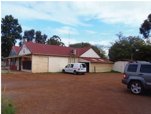
Post Office, Northern Side View
