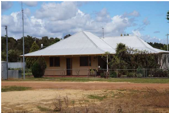
Front elevation, looking south east
