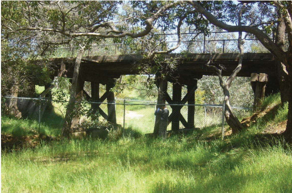
Railway Bridge view east to west – Source: Stephen Carrick Architects, conservation plan, 2014 (SJ1-01 pic 1)
