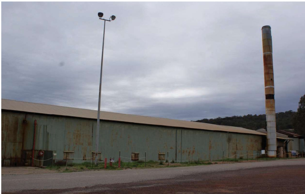
Kiln Shed, View north east – Source: Austral Bricks, 2022 (SJ2-03 pic 1)
