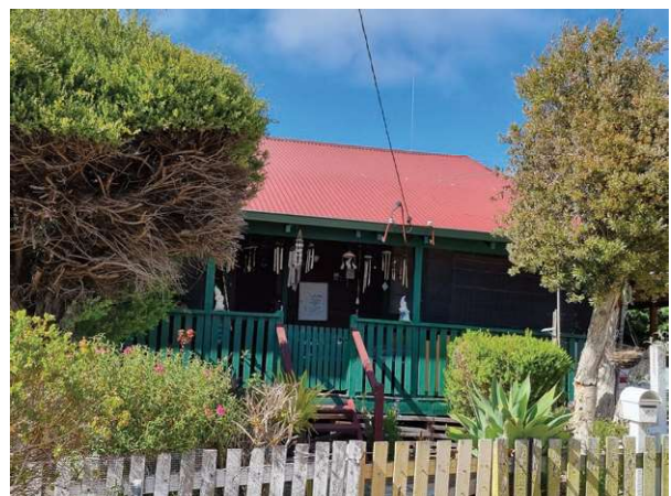
Source: Shire of Serpentine Jarrahdale, 2022 (SJ5-14 pic 5)
