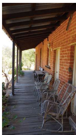
Verandah (East looking West)
