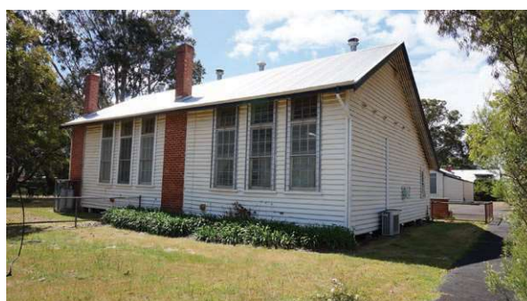
Mundijong School 1st building (fmr), Southern Side
