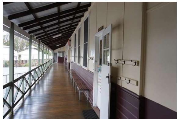
Verandah looking East
