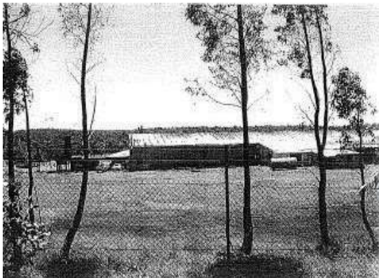
Previous Local Heritage Survey, 2000 Source: Shire of Serpentine Jarrahdale (SJ5-11 pic 3)
