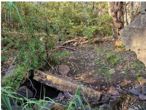
Dam wall within the brook, Source: Shire of Serpentine Jarrahdale, 2022 (SJ5-16 pic 4)
