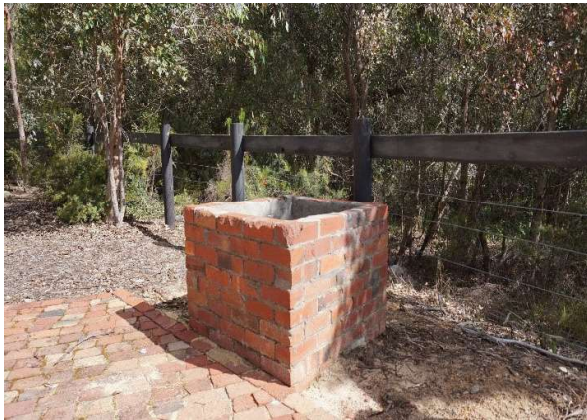
View South East
