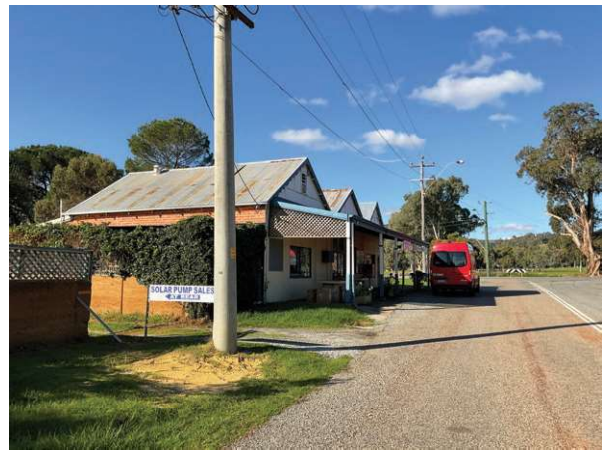
Keysbrook General Store, Front Verandah, West view to East
