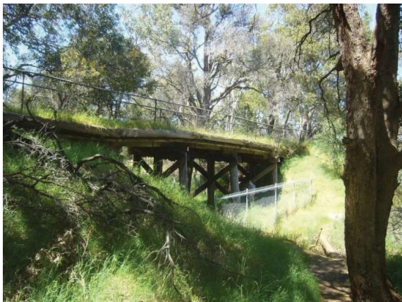
Brickworks Railway Bridge, view looking South East Source: Stephen Carrick Architects 2014 (SJ1-01 pic 4)
