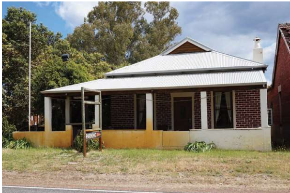
Front elevation of Left house
