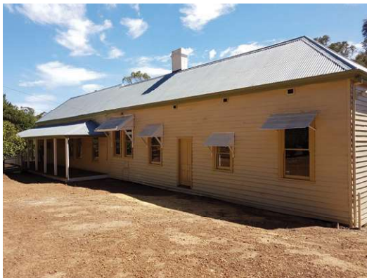
Mill Manager's Residence, South East looking North West
