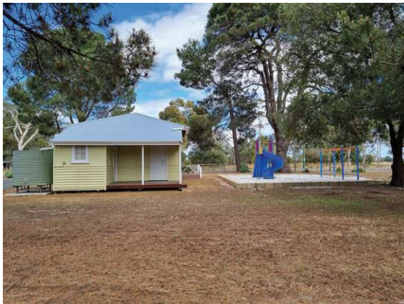
Rear elevation including playground
