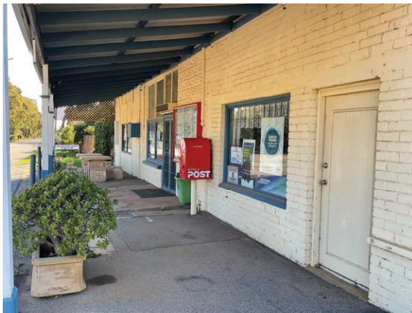
Keysbrook General Store, Front Verandah, East view to West
