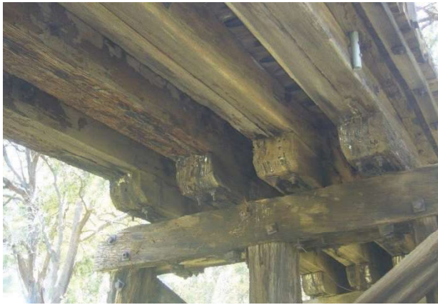
Brickworks Railway Bridge, underneath Source: Stephen Carrick Architects 2014 (SJ1-01 pic 2)
