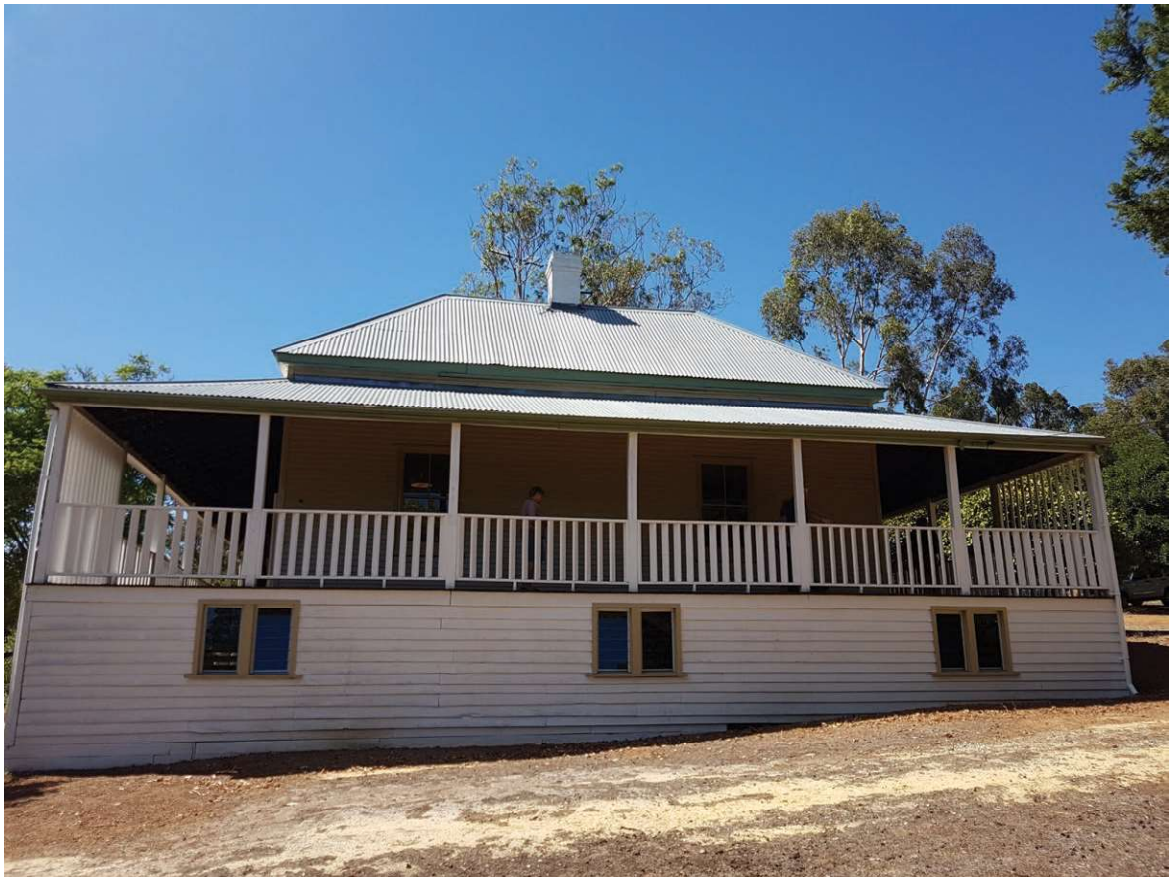
Mill Manager's Residence, View West to East – Source: Shire of Serpentine Jarrahdale, 2020 (SJ5-10 pic 1)
