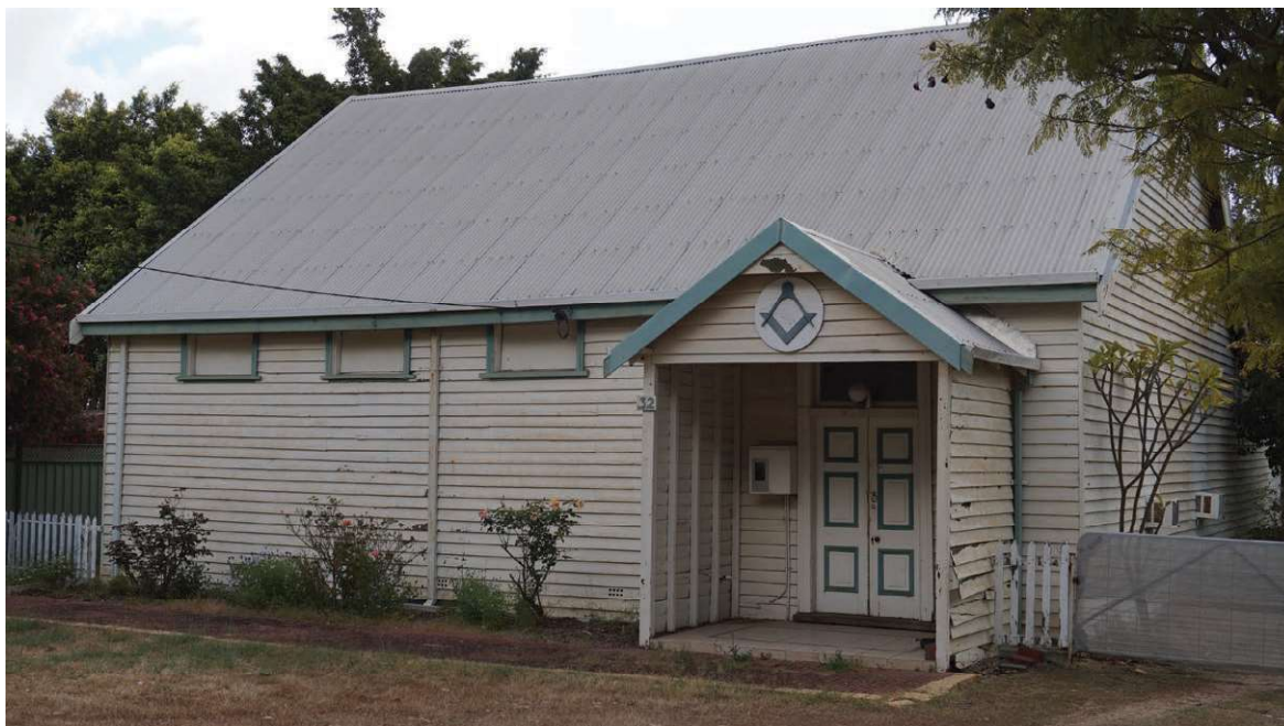
Front View, looking West – Source: Shire of Serpentine Jarrahdale, 2022 (SJ9-09 pic 1)
