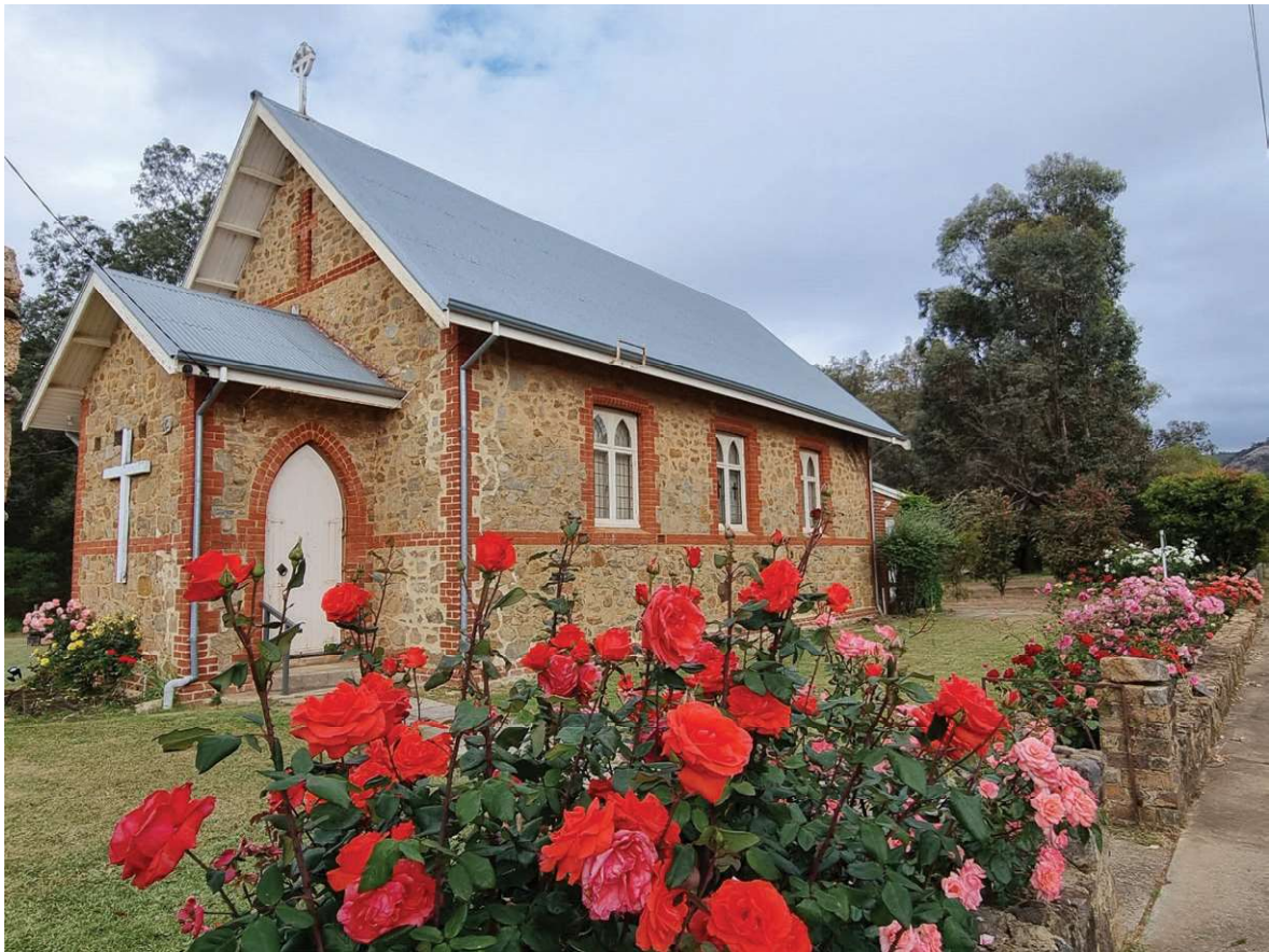
St Stephen's Church, front/side elevation, viewing the rose gardens and Baldwin's Bluff in the background. Source: Shire of Serpentine Jarrahdale, 2022 (SJ12-01 pic 1)
