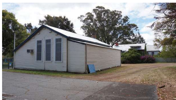
Mundijong School 2nd building (fmr), Southern Side View
