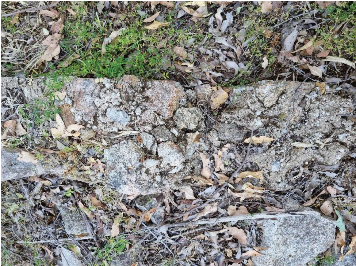
Waterwheel house cornerstone, Source: Shire of Serpentine Jarrahdale 2022 (SJ5-16 PIC 1)
