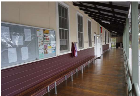
Verandah looking West
