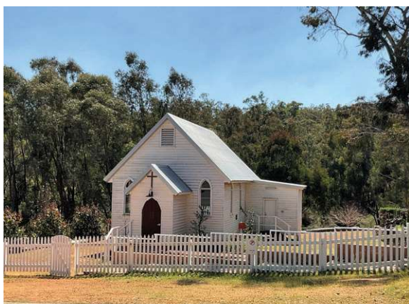
Front View North/West
