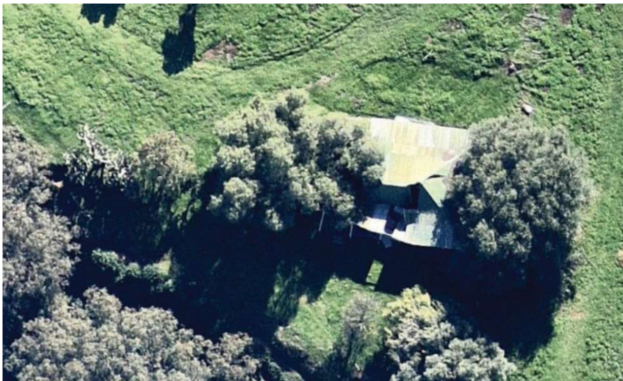
Aerial view – Shire of Serpentine Jarrahdale, 2022 (SJ12-16 pic 1)
