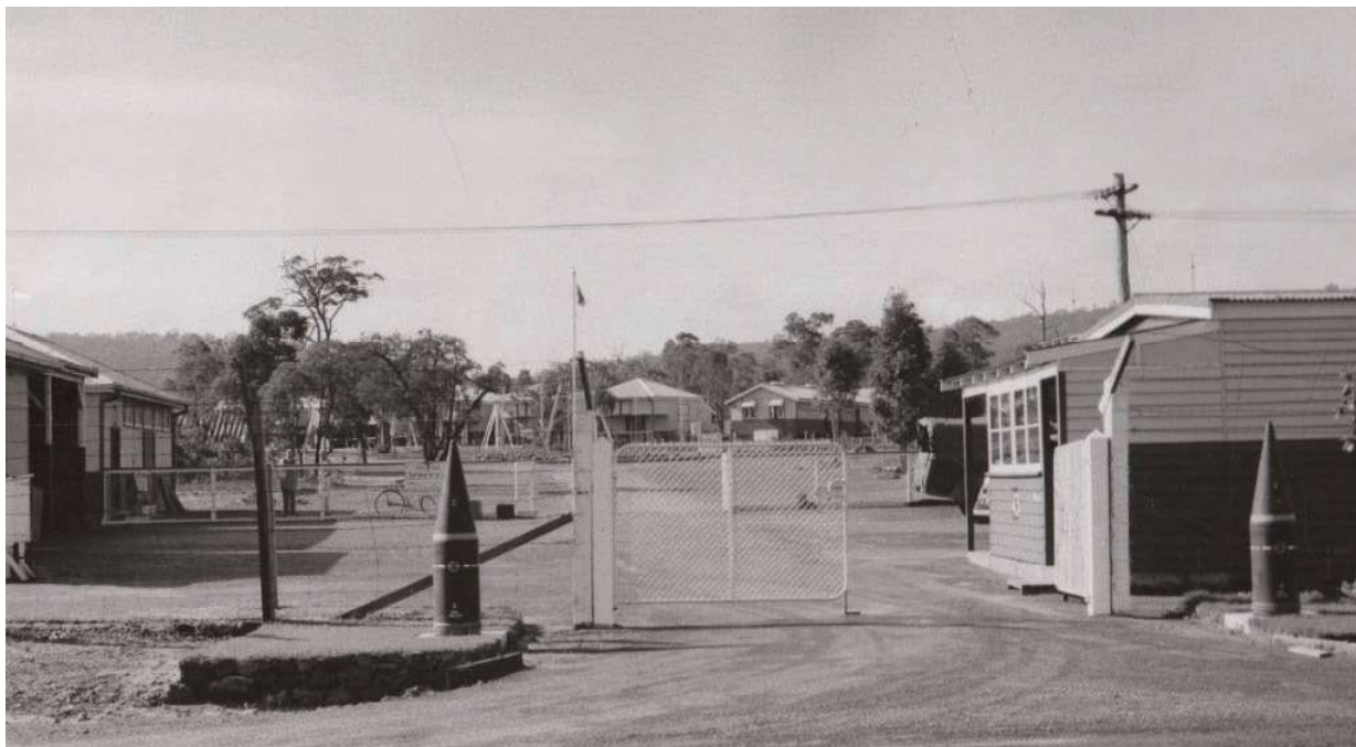
Byford Main entrance to Depot – Source: SLWA_b3526926_4 (SJ1-06 pic 1)
