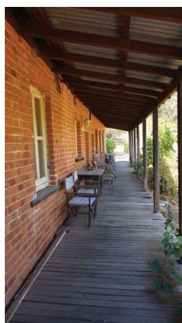
Verandah (West looking East)
