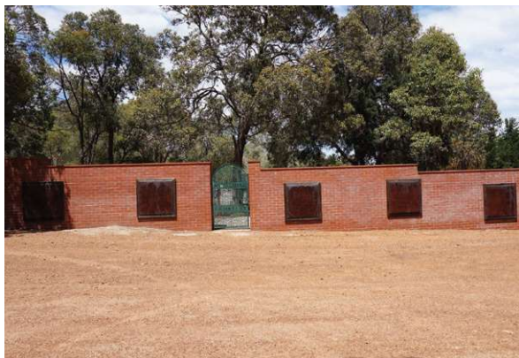
Source: Shire of Serpentine Jarrahdale, 2022 (SJ12-07 pic 2)
