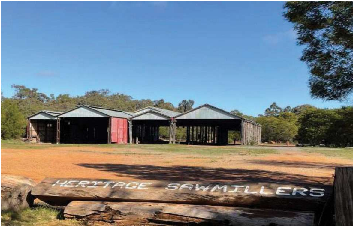
Mill Sheds – Source: Stephen Carrick Architects, 2022 (SJ5-01 pic 1)
