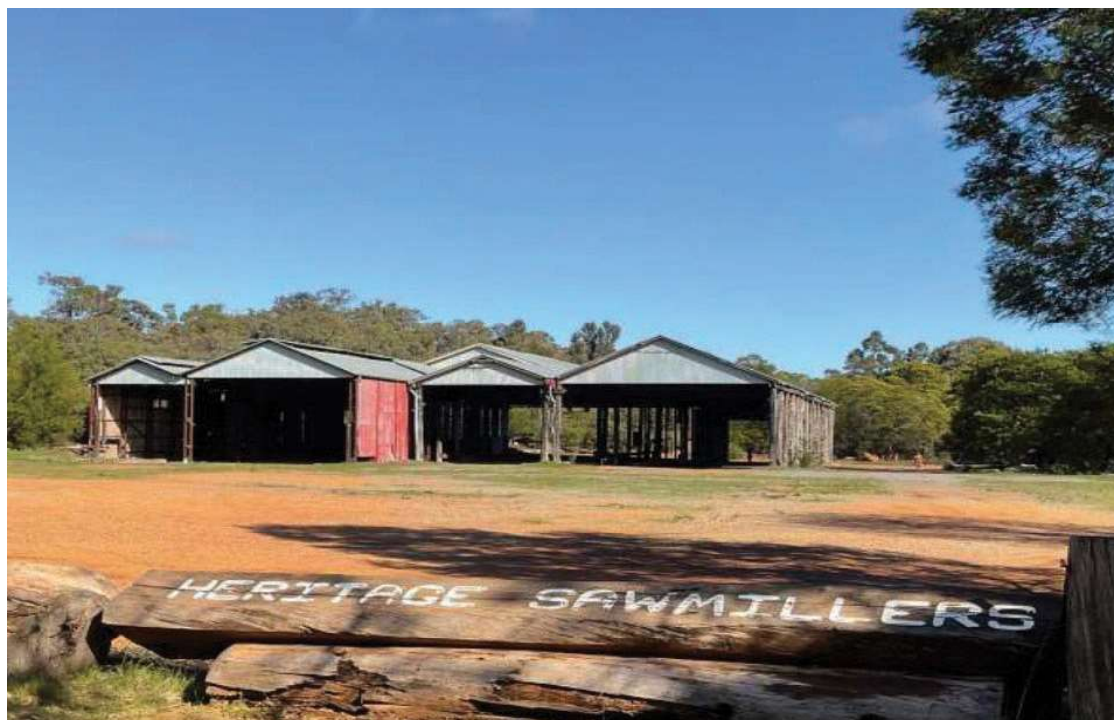
Mill Sheds – Source: Stephen Carrick Architects, 2022 (SJ5-11 pic 1)
