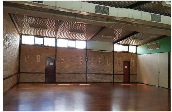
Interior, looking North
