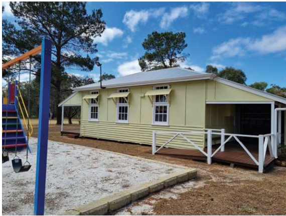
Side view (north)
