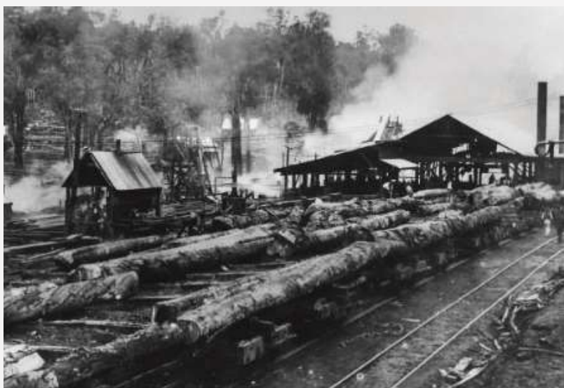
Figure 1 Jarrahdale Timber Milling 1900–1910 (SLWA 1458b1–5A 014738 PD)
