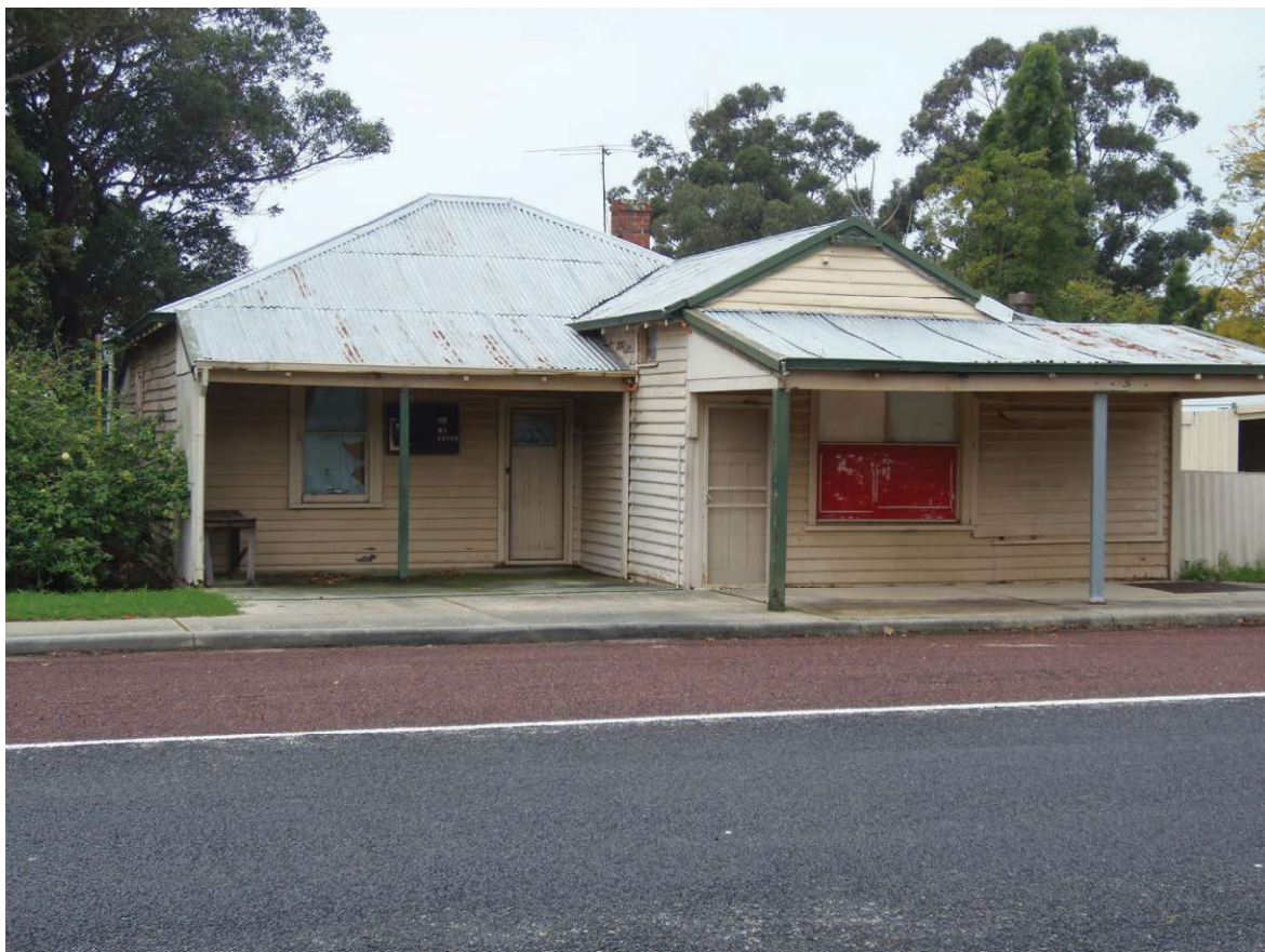
Wellard Street view – Source: Stephen Carrick Architects, 2022 (SJ12-23 pic 1)
