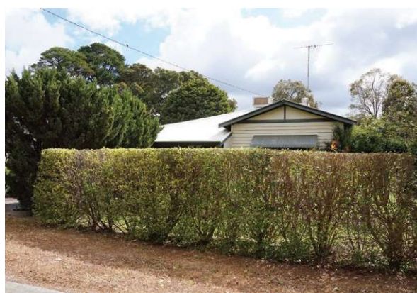
Source: Shire of Serpentine Jarrahdale, 2022 (SJ5-13 pic 3)
