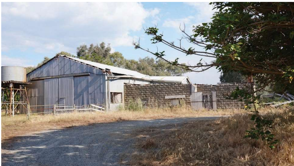
Side elevation, looking South – Source: Shire of Serpentine Jarrahdale, 2022 (SJ2-04 pic 1)
