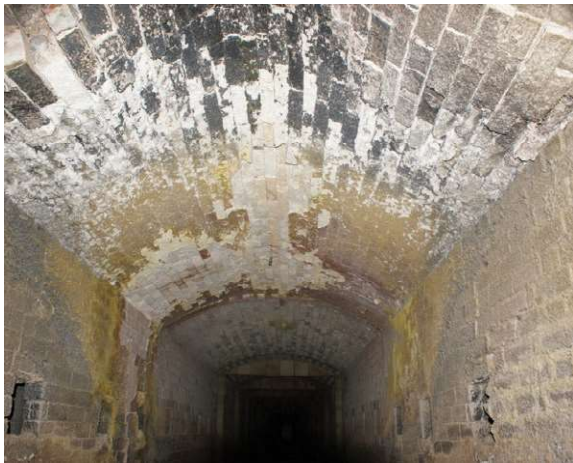
Kiln Interior, View East
