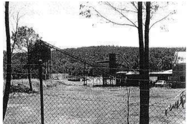
Previous Local Heritage Survey, 2000 Source: Shire of Serpentine Jarrahdale (SJ5-11 pic 4)
