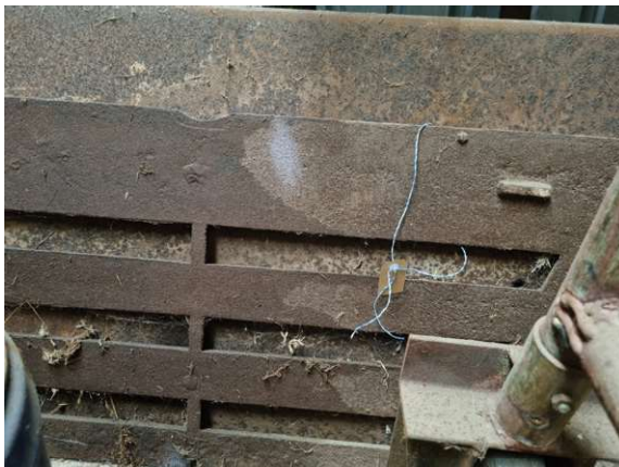
Source: Shire of Serpentine Jarrahdale, Fire grate (SJ1-10 PIC 4)
