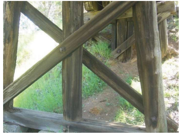
Brickworks Railway Bridge, Underneath pylons and cross beams Source: Stephen Carrick Architects 2014 (SJ1-01 pic 3)
