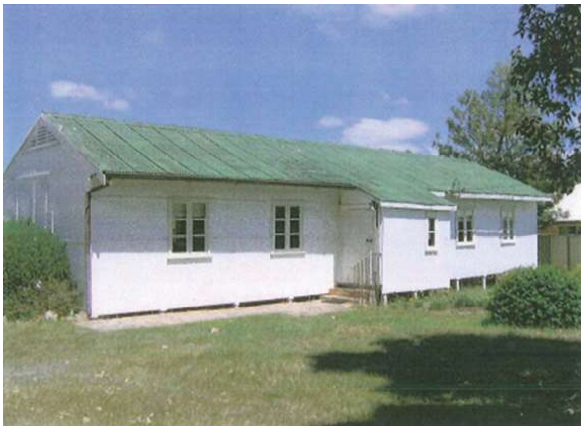
Front elevation, Clifton Street – Source: Shire of Serpentine Jarrahdale, 2008 (SJ1-03 pic 1)
