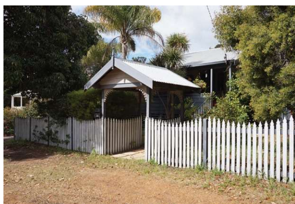
Source: Shire of Serpentine Jarrahdale, 2022 (SJ5-13 pic 2)
