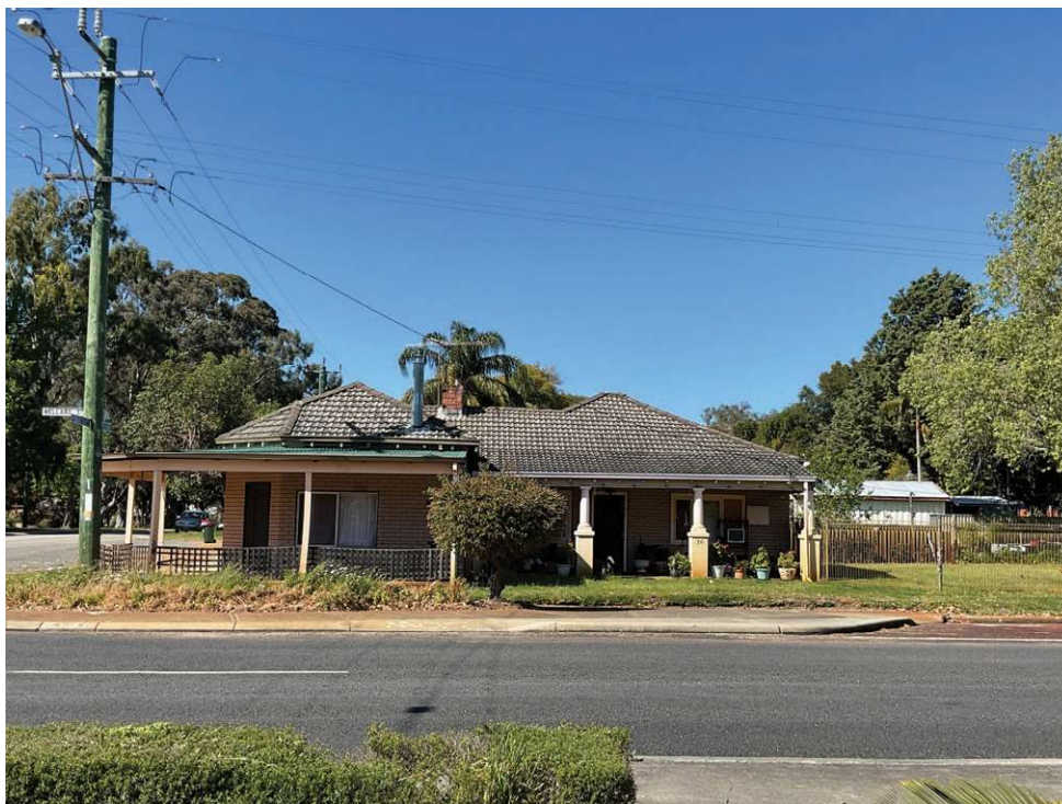
Wellard Street view – Source: Stephen Carrick Architects, 2022 (SJ12-26 pic 1)
