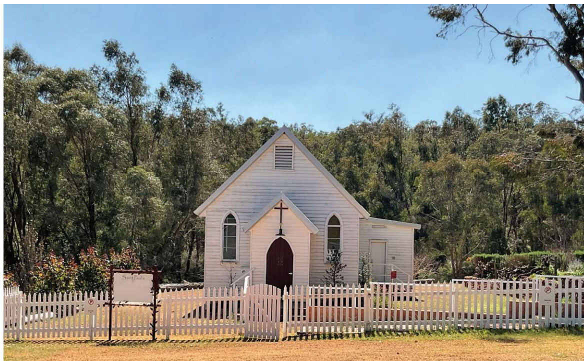
St. Paul's Church – View North – Source: Stephen Carrick Architects, 2022 (SJ5-03 pic 1)
