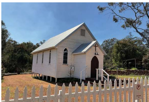
Front View North East
