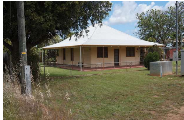
Front elevation, looking south west
