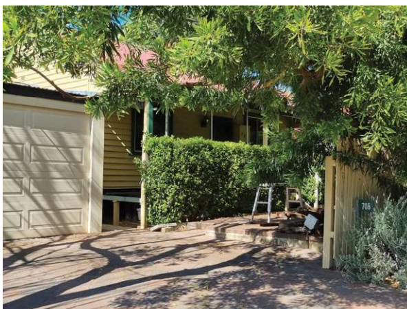
Source: Shire of Serpentine Jarrahdale, 2022 (SJ5-14 pic 4)
