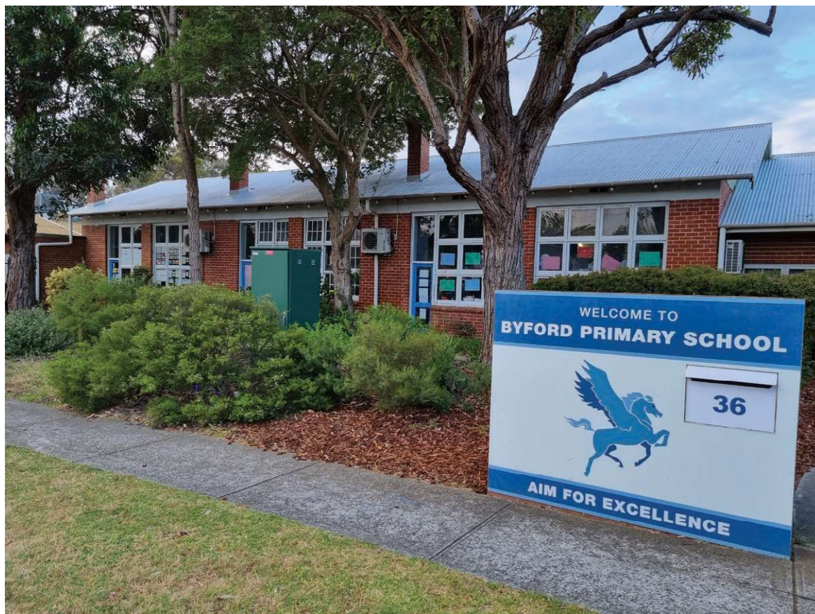
Front elevation, Clifton Street – Source: Shire of Serpentine Jarrahdale, 2022 (SJ1-14 pic 1)
