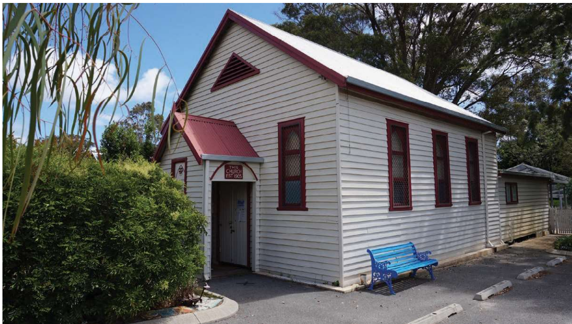
Uniting Church, Front View – Source: Shire of Serpentine Jarrahdale, 2022 (SJ9-01 pic 1)
