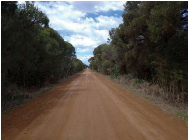
Source: Shire of Serpentine Jarrahdale, 2022 (SJ15-03 pic 4)
