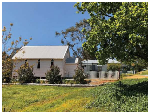
Side View East
