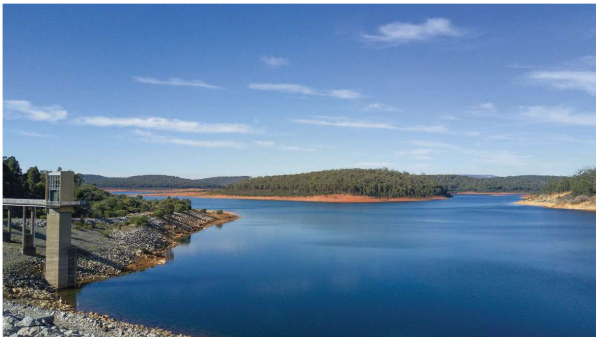
Serpentine Dam Wall view over water body and tower, 2020 – Source: Shire of Serpentine Jarrahdale (SJ12-21 pic 1)
