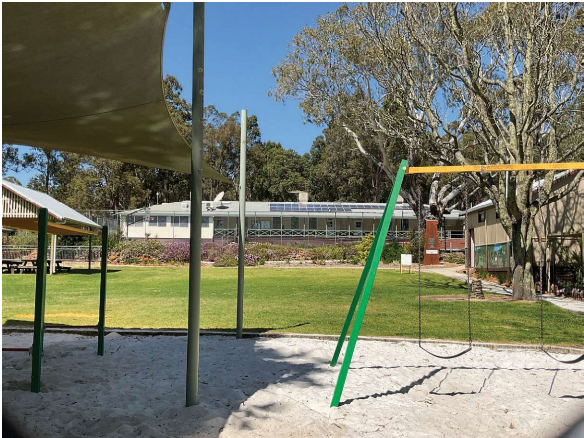
View from Wanliss Street – Source: Stephen Carrick Architects, 2022 (SJ5-08 pic 1)
