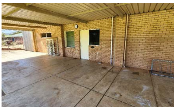
Drainage I.O's Visible on Slab
