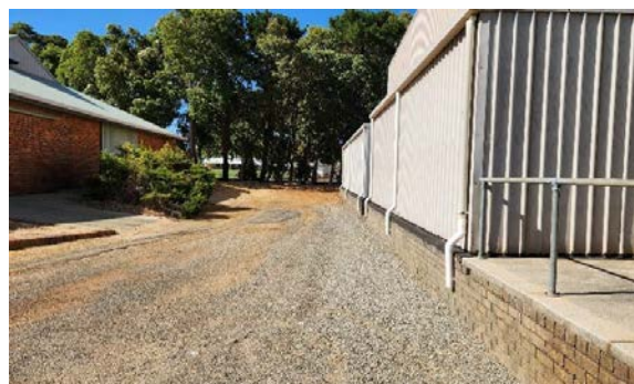
Storeroom Roof Downpipe Discharging on Ground Level
