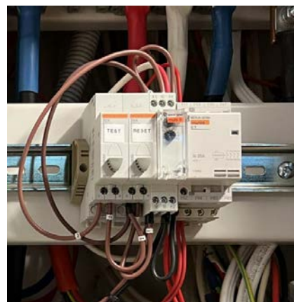
Emergency Lighting Test Switch
