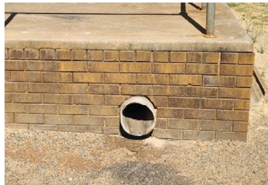
Stormwater Overflow Pipe Under Lean-to Structure
