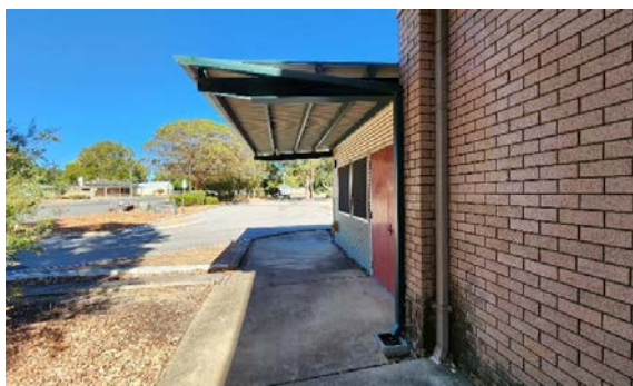
South Elevation Downpipe Connecting In-ground
