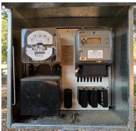
Pole Mounted Meter Box
