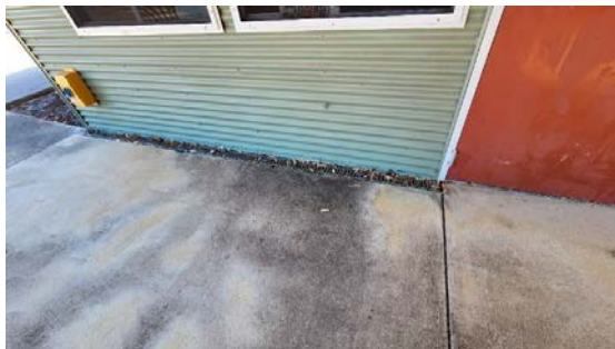
Lean-to Roof Downpipe Discharging on Ground Level
