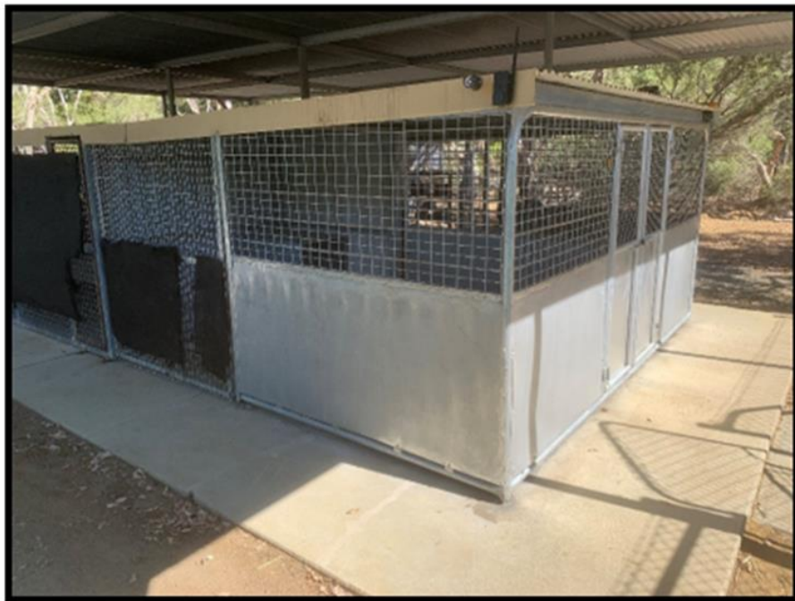
The Shire Pound enclosure shaded by second roof structure
