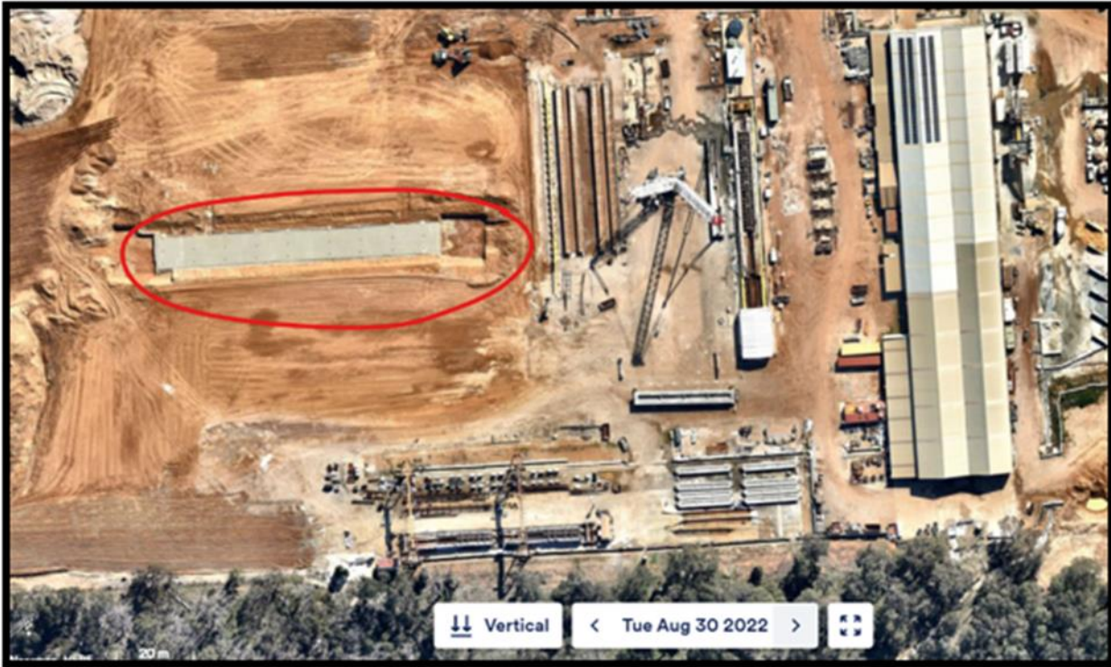
30 August 2022. Note new stressing bed being built with no Shire or DWER approval. Located close to the western boundary, and orientated in such a way that noise is directed in an east west direction
