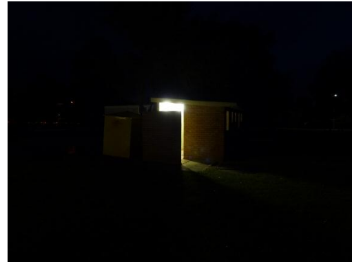
Figure 6: View West Female Entrance to Ablution Block - Night
