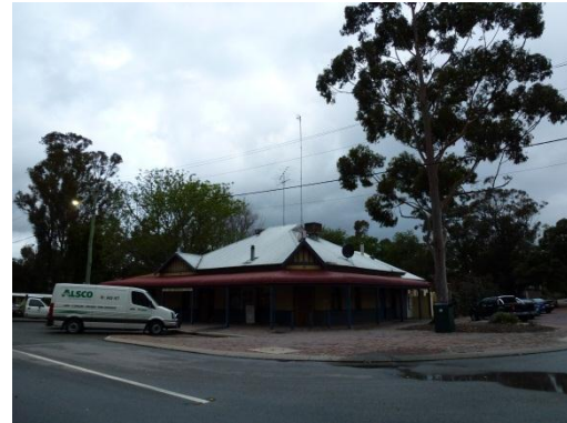
Figure 36: Clear sightlines at entrance to licensed premises enhance natural surveillance and community safety perceptions
