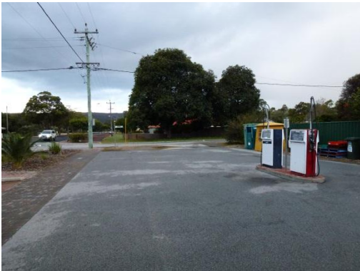
Figure 27: Climbing debris and natural ladders located adjacent fencing providing opportunity for offenders. Good natural surveillance adjacent petrol pumps
