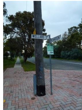
Figure 38: Signage appears damaged and requires rectification
