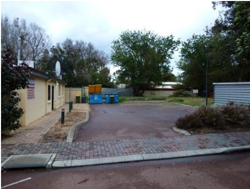
Figure 35: Area requires maintenance to enhance a sense of ownership for the community and deter potential offenders from congregating in the area
