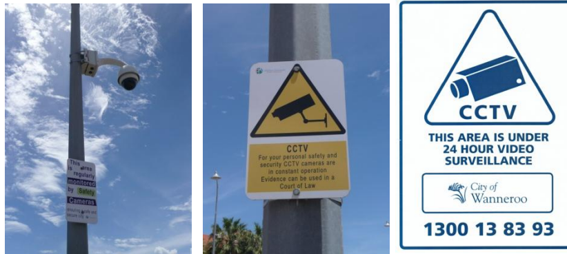
Figure 5: Samples of CCTV Signage and Pole Mounting
