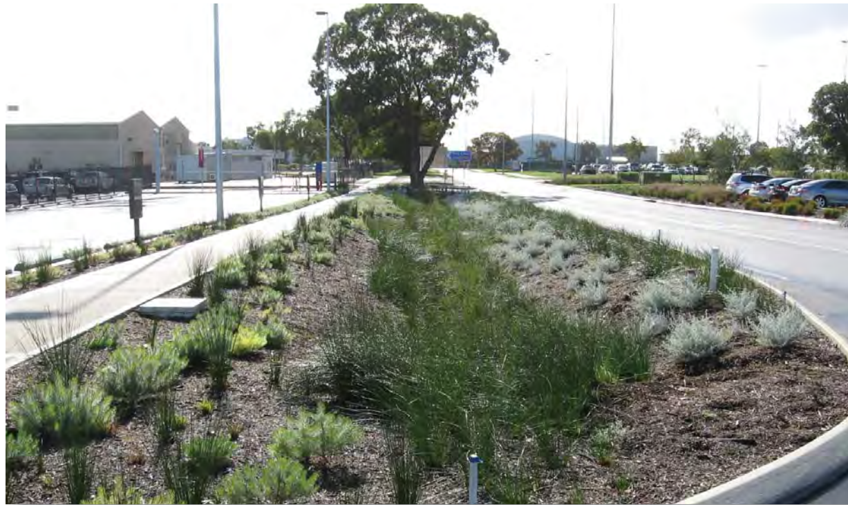
Bio Swale Example - Perth Airport
