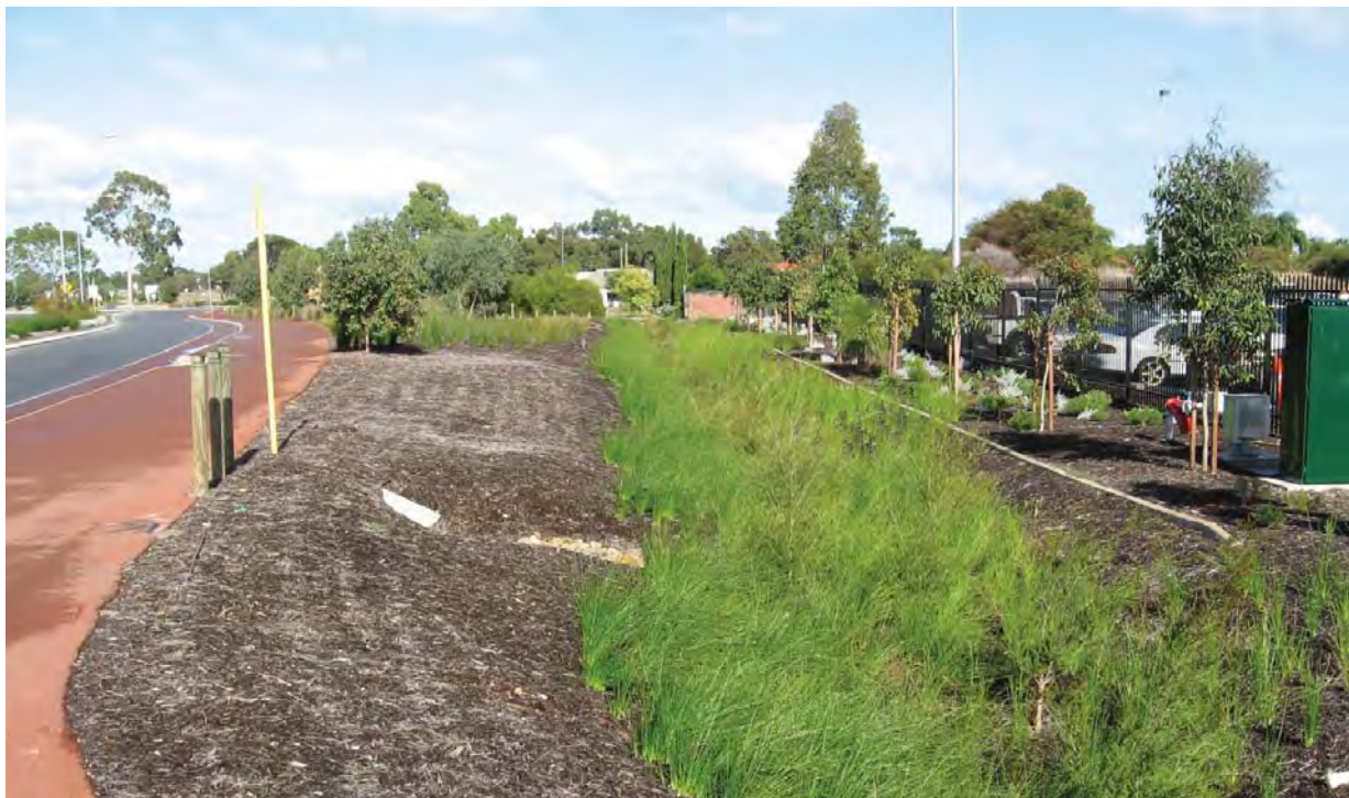
Bio Swale Example - Perth Airport
