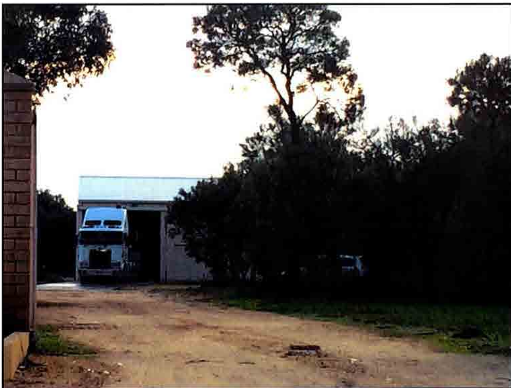
Photo 4: An example of a shed within the immediate locality which is visible from the street
