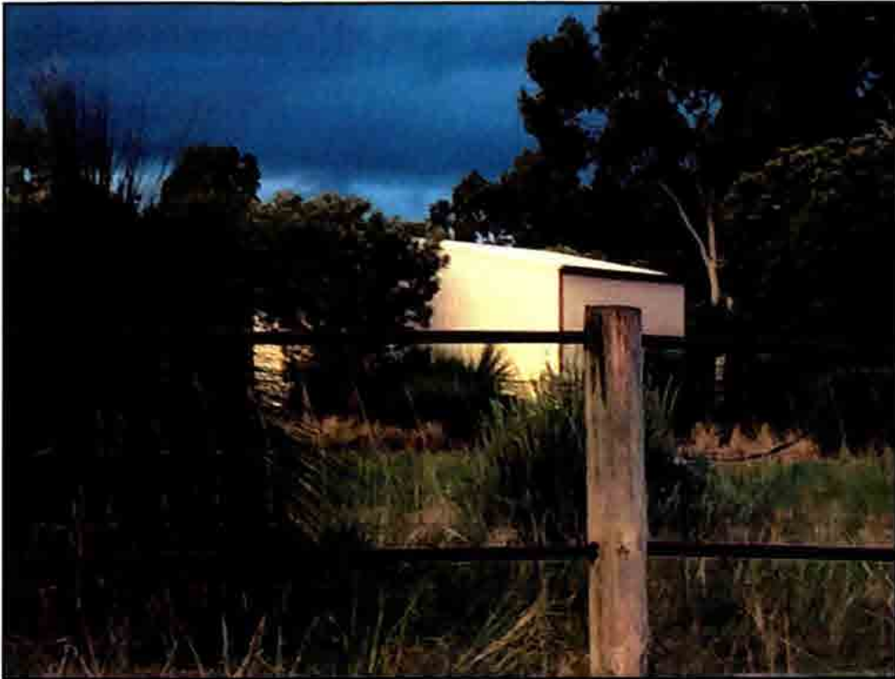
Photo 3: An example of a shed within the immediate locality which is visible from the street
