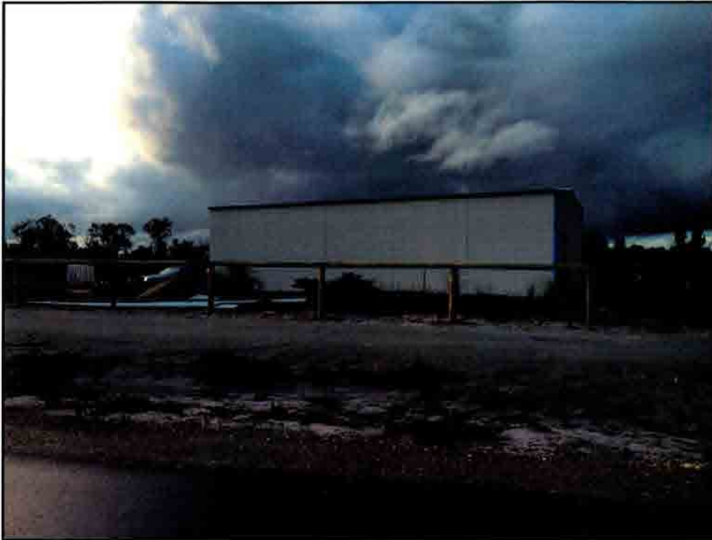
Photo 5: An example of a shed within the immediate locality which is visible from the street
